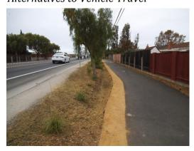
The multi-modal pathway was installed along this roadway utilized recycled (reclaimed) asphalt concrete pavement in its construction. Separated from the main roadway by a landscaping, the pathway offers an alternative for the casual cyclist or pedestrian wanting to walk or cycle along this busy roadway. A 2' wide gravel pathway was also installed adjacent to this pathway and provides a separate place for runners.
