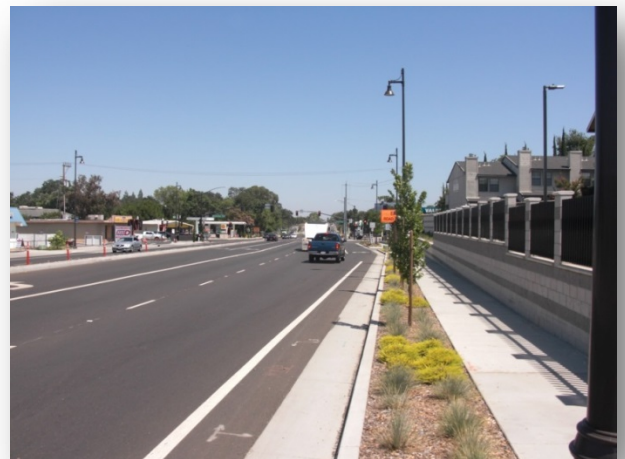
Figure 6-After Construction with Landscaping Buffer for Sidewalk, Dedicated Class II Bike Lane and Raised Median
