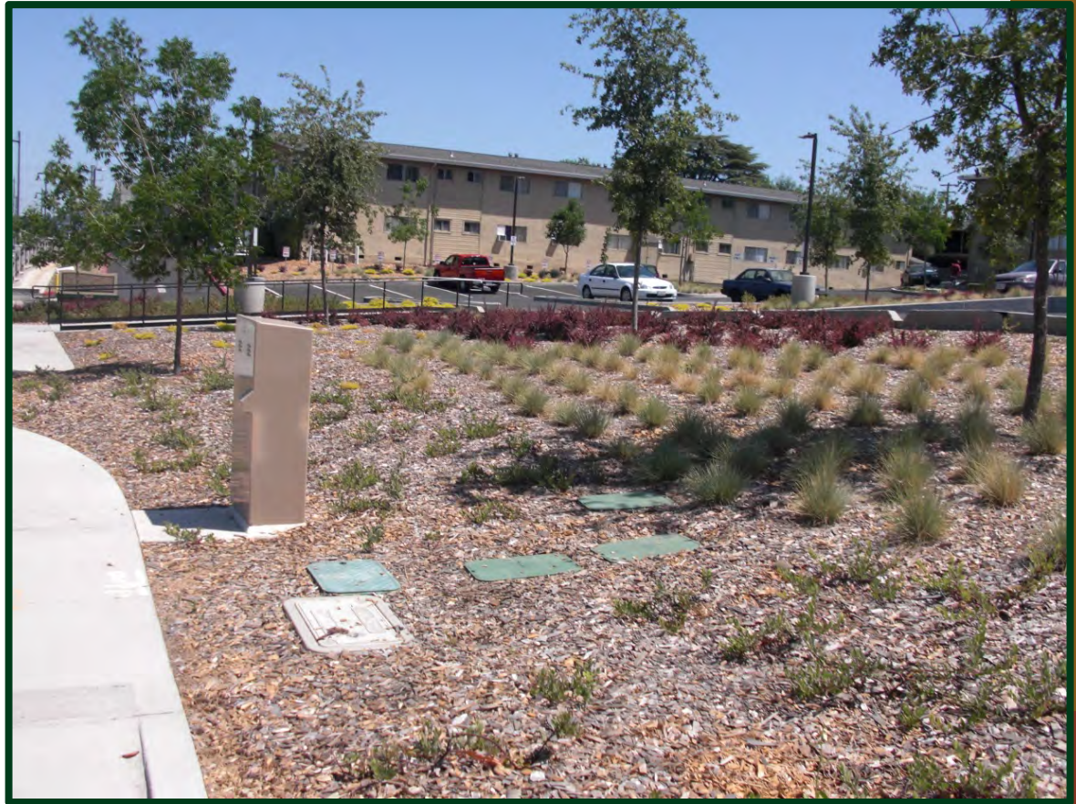
After: Parking lot for Sierra Oaks Apartments
