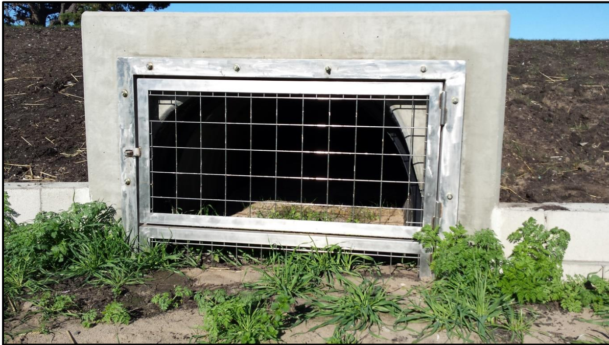
. Specialized metal grates cover the opening to the pipe to keep other varmints from eating salamanders in the pipe.
