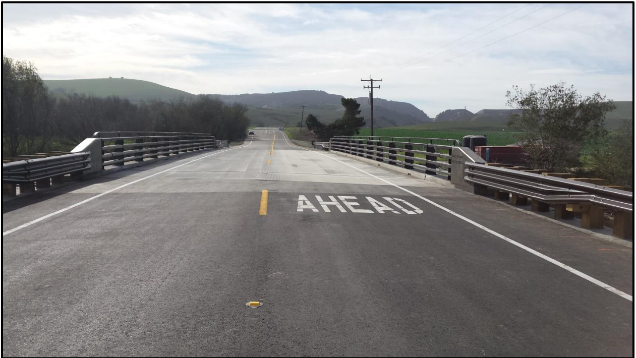
The new bridge is a strong 94-foot, 38-foot wide superstructure, with two 12-foot lanes, two 5-foot shoulders, and two 2-foot wide sustainable guardrail elements on the deck.
