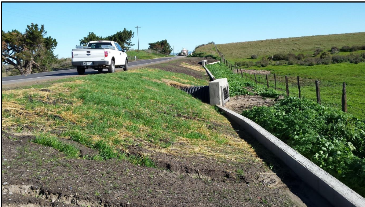
Low-lying walls encourage salamanders to move to a central pipeline to convey them beneath the road
