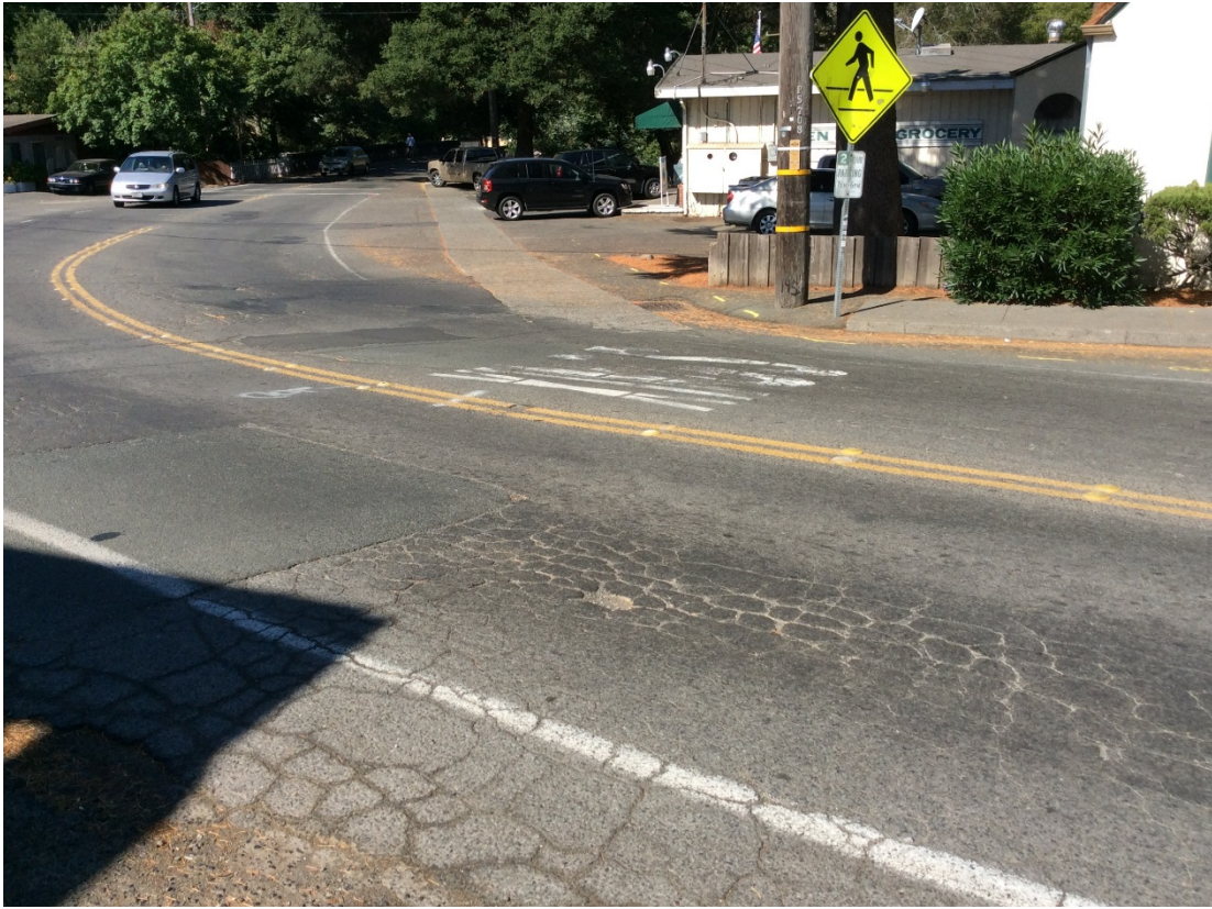
Location Four, Before and After
