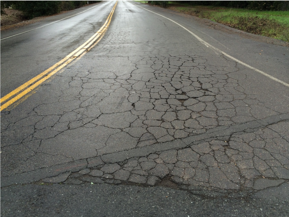
Location Five, Before and After
