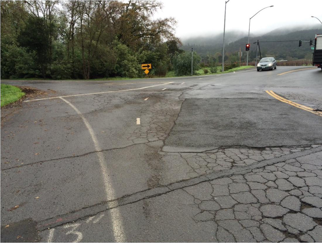
Location Two, Before and After
