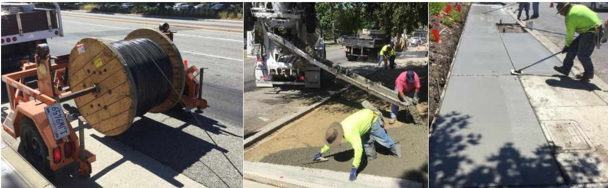
Figure 10 - Examples of Phase 3 Construction Activities
