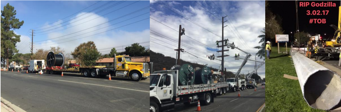
Figure 9 - Examples of Phase 2 Construction Activities
