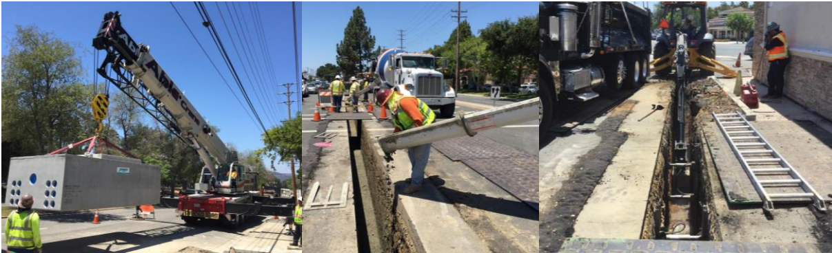
Figure 8 - Additional examples of Phase 1 construction activities
