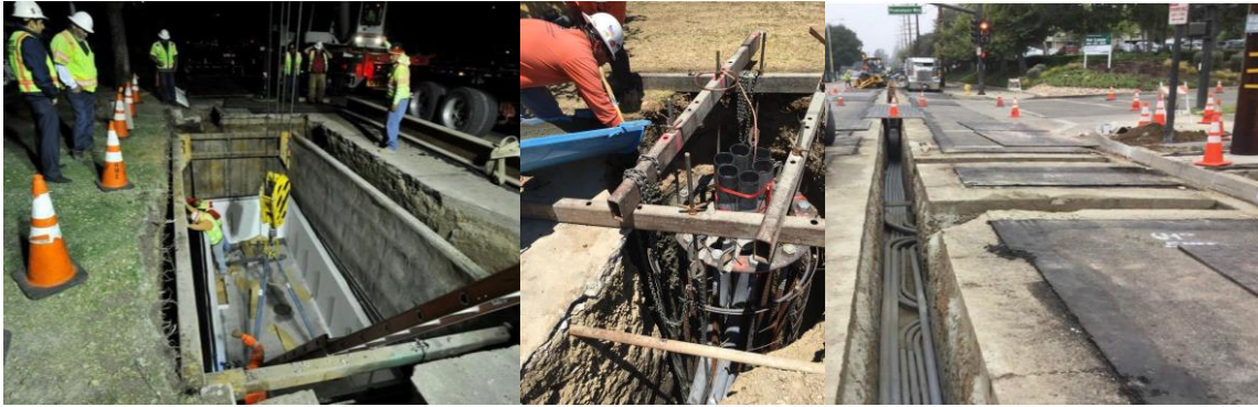
Figure 7 - Examples of Phase 1 construction activities
