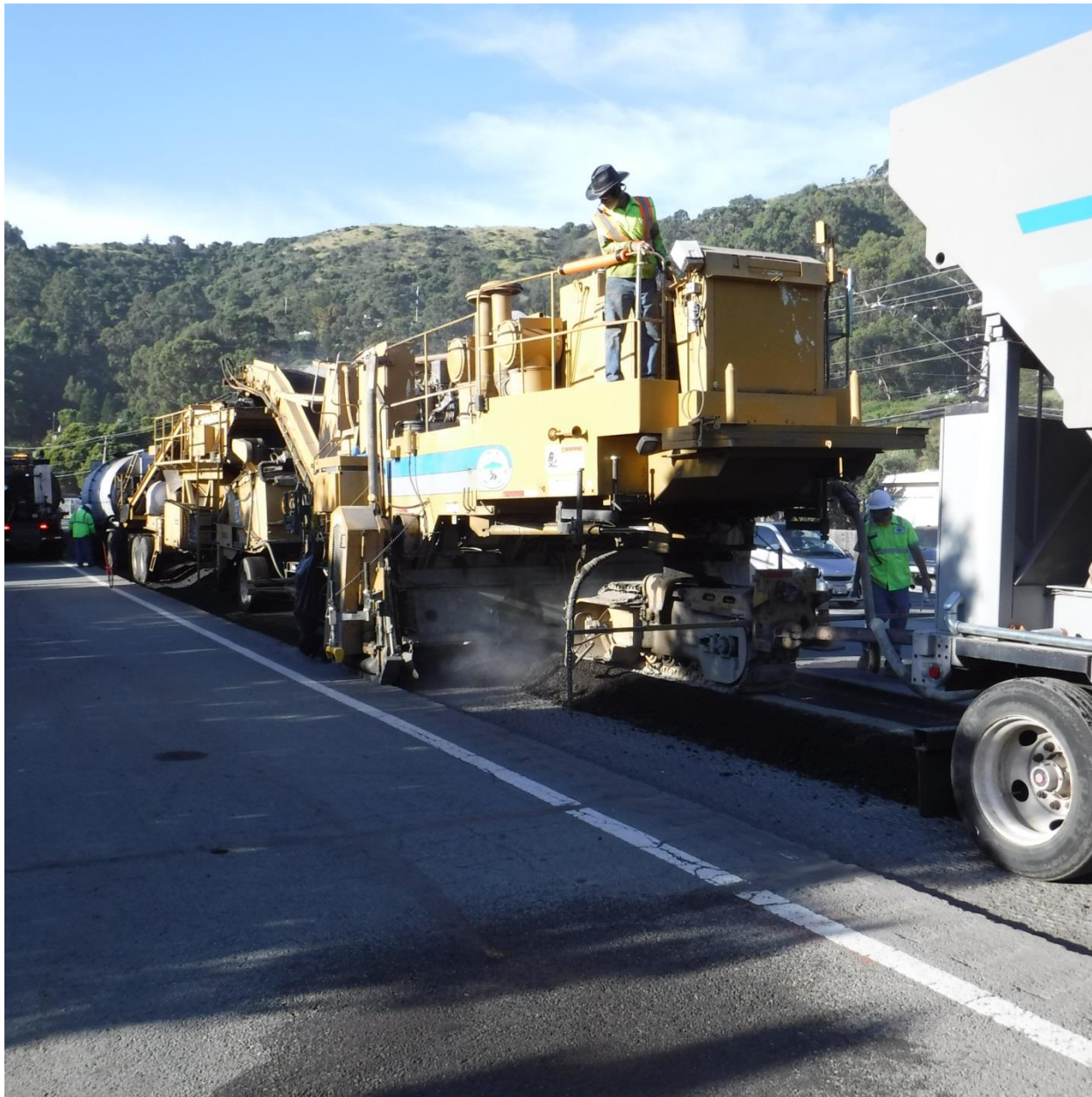
Cold-In-Place recycling train
