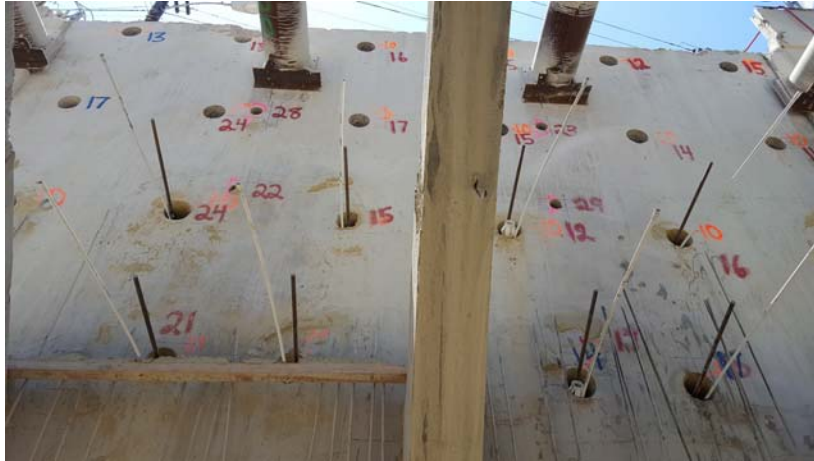
Installation of Remaining Ground Anchors
