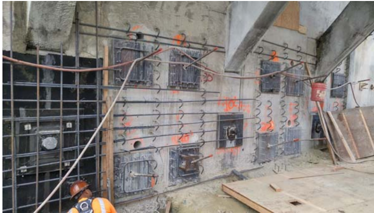
Abutment New Facing Construction
