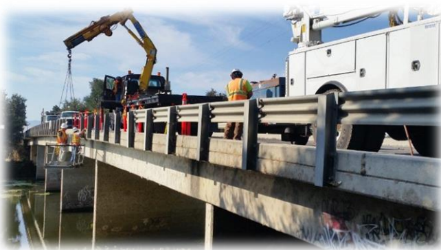
Figure 1: Left: County crew performing bridge inspection with a boom truck. Right: County drone approaching truss of bridge for inspection of structural members.
