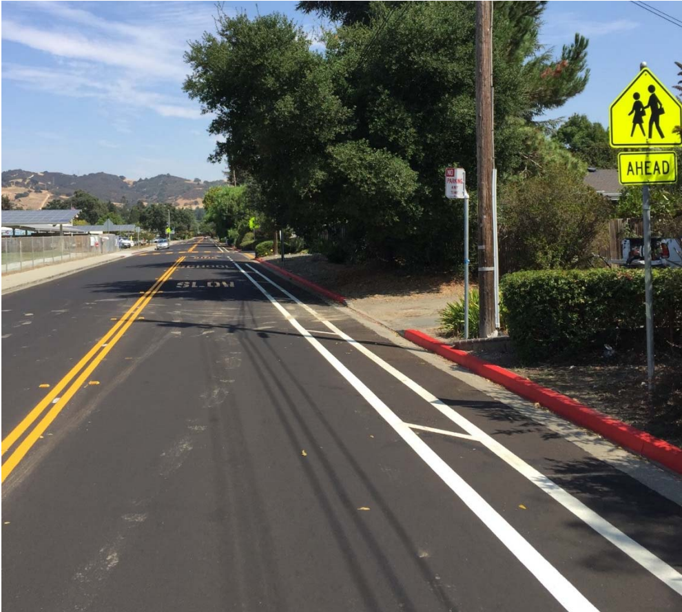
After Construction: Cedro Lane
