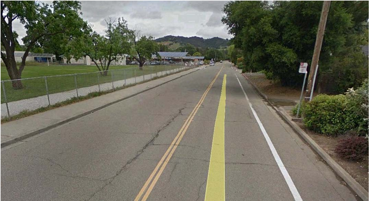
Before Construction: Cedro Lane
