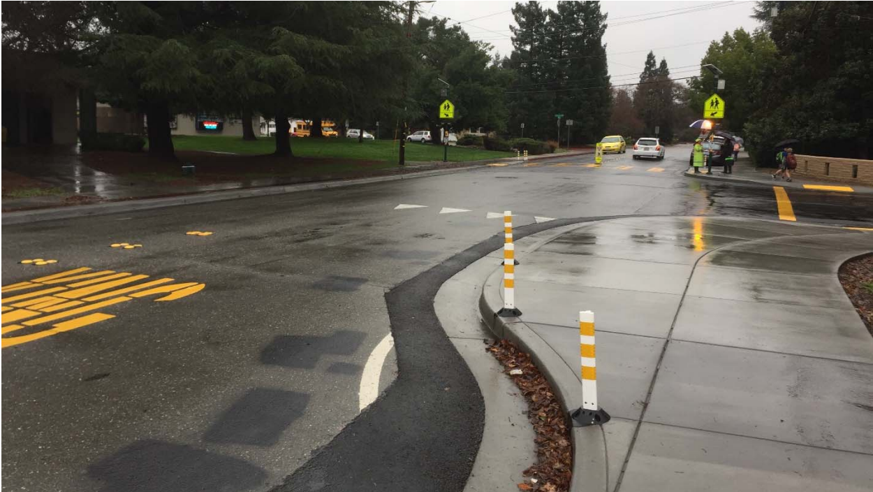
After Construction: Wiget Lane & Blackstone Drive
