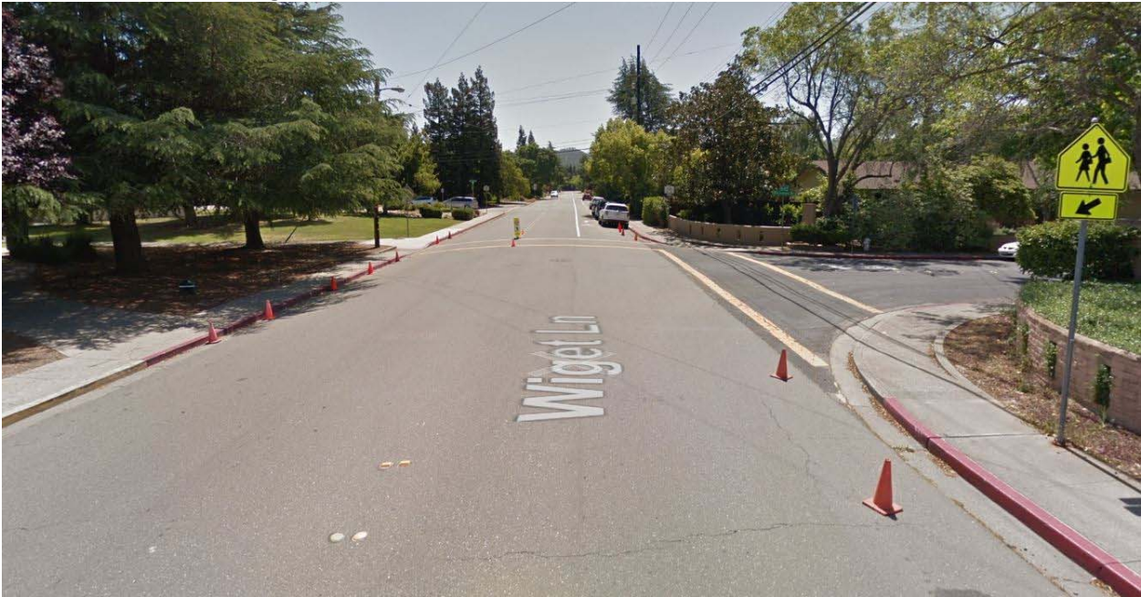
Before Construction: Wiget Lane & Blackstone Drive
