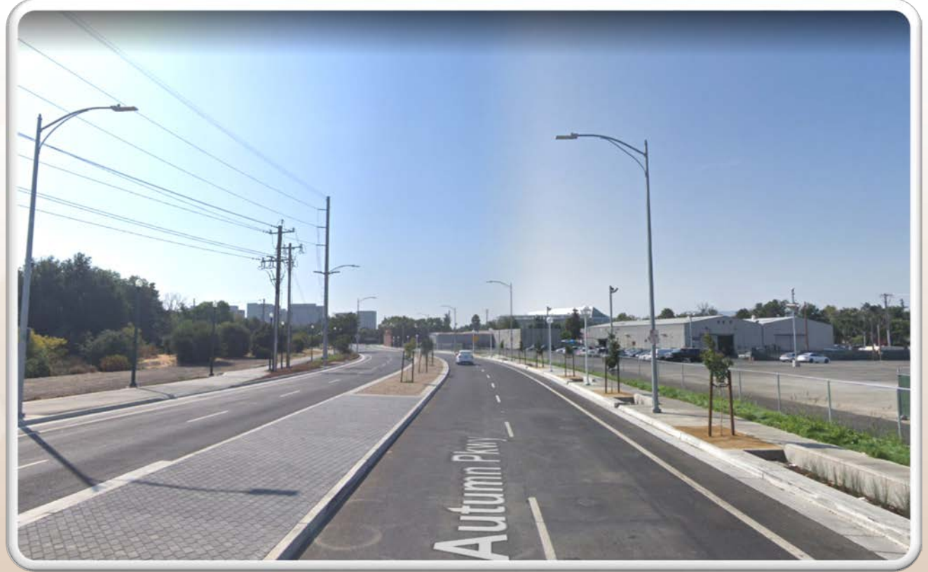
New Autumn Parkway looking south
