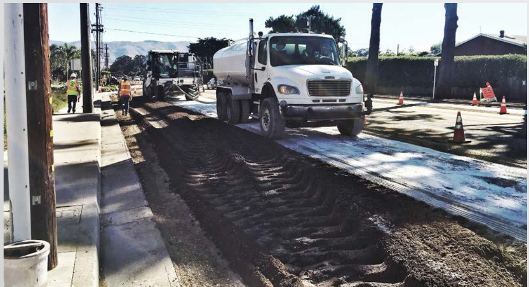
Lime treatment of existing material during full depth reclamation process
