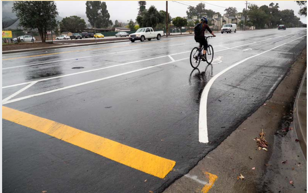
Microsurfacing and buffered bike lane
