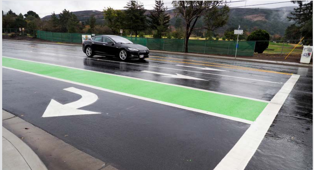
Microsurfacing and green bike lane
