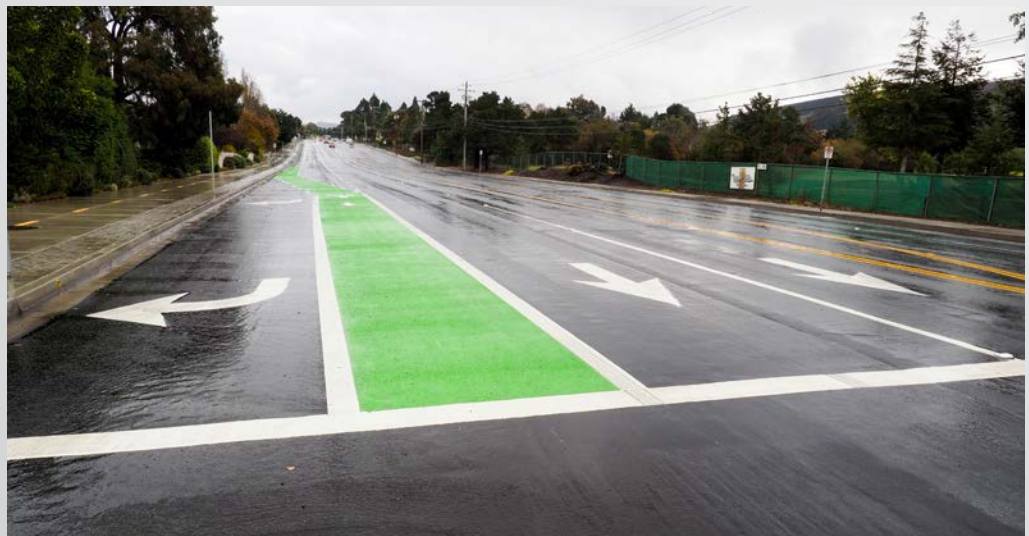
Microsurfacing and green bike lane
