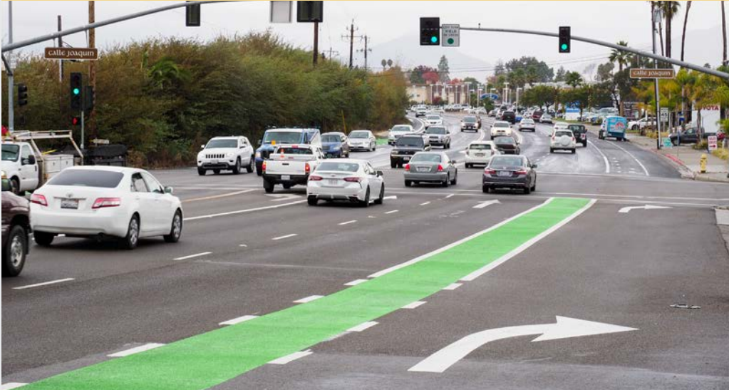
Microsurfacing and green bike lane
