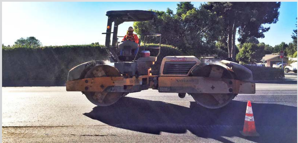
Pavement compaction of new asphalt
