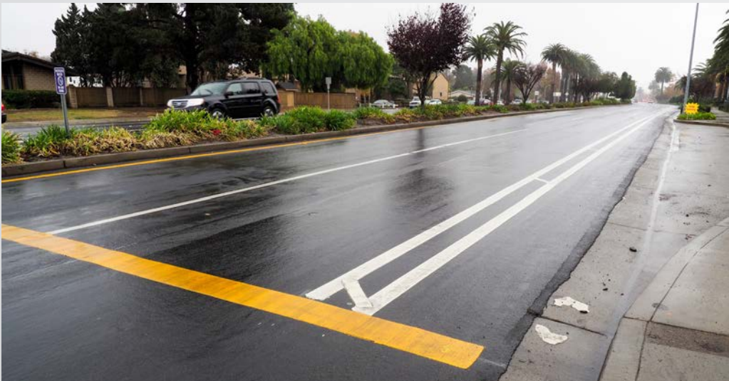
Microsurfacing and buffered bike lane
