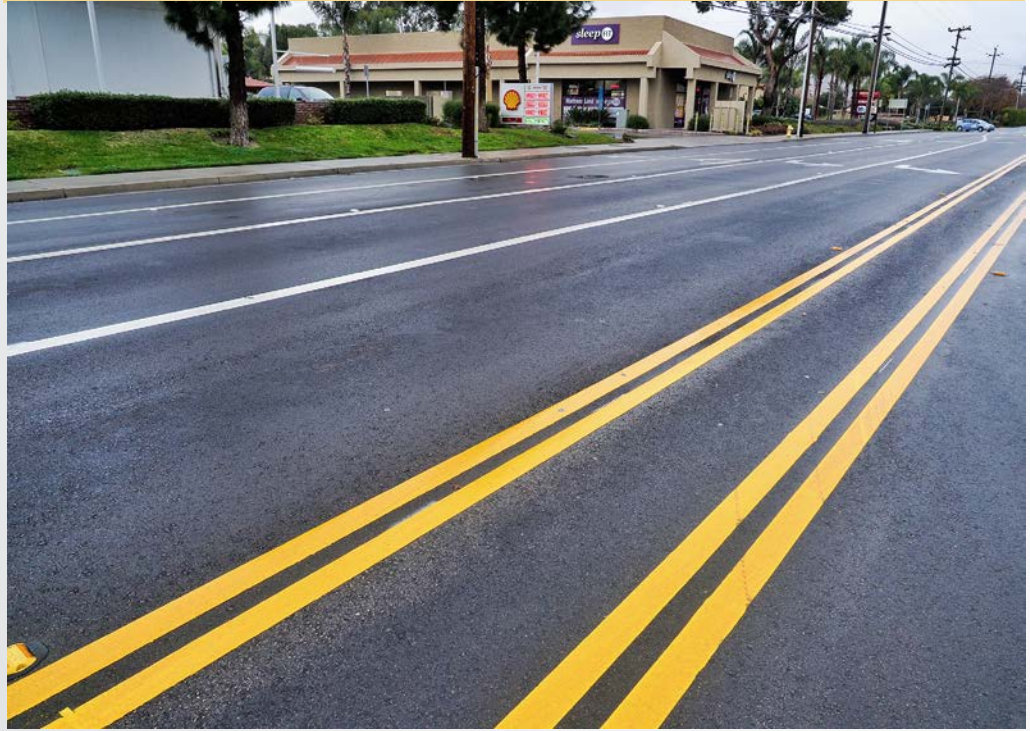
Finished asphalt pavement and fresh striping of FDR treated area
