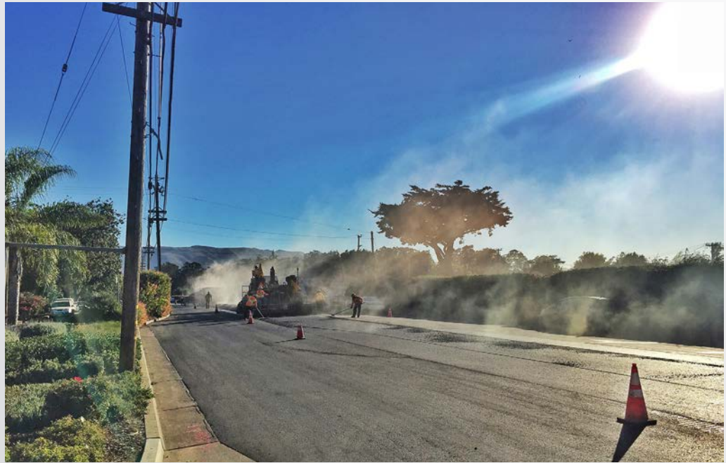
Paving over the FDR treated subgrade
