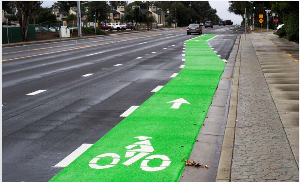
Microsurfacing and green bike lane at vehicle crossing zone
