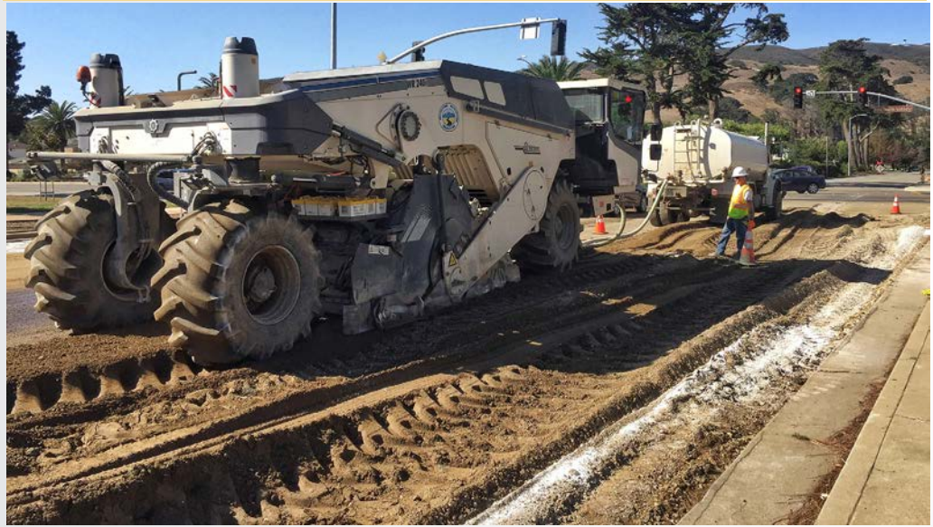
Pulverization and mixing of in-place material during full depth reclamation process
