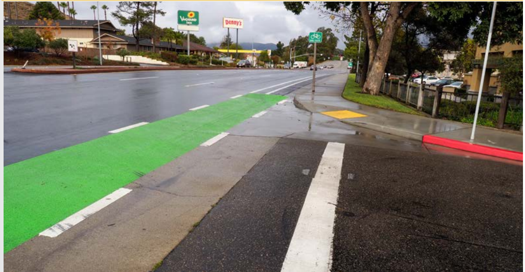
Microsurfacing and green bike lane at vehicle crossing zone
