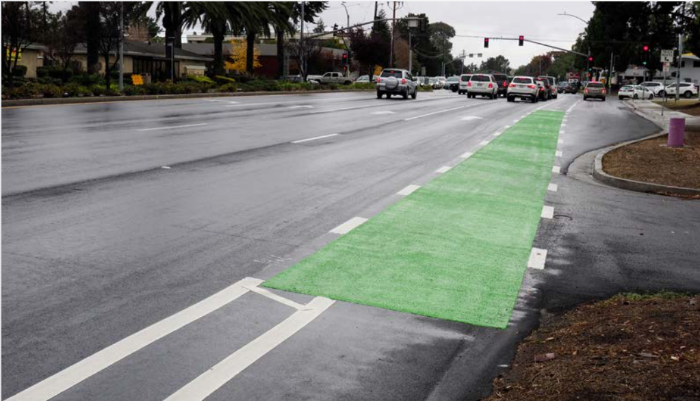
Microsurfacing and green bike lane at vehicle crossing zone
