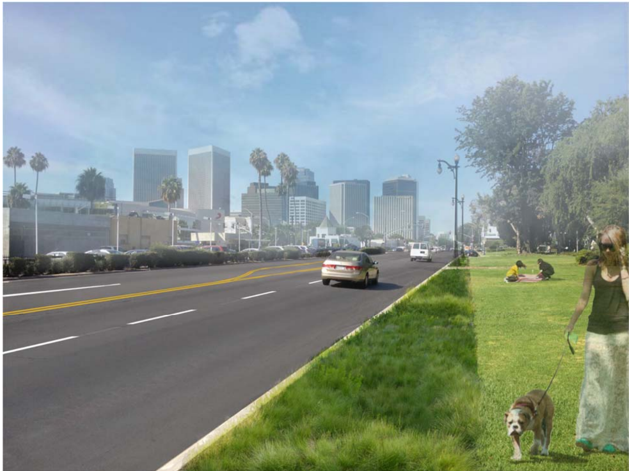
Figure 1: Complete Street- Bioswale, LED Lighting, Road Reconstruction, Recycled Water Irrigation
