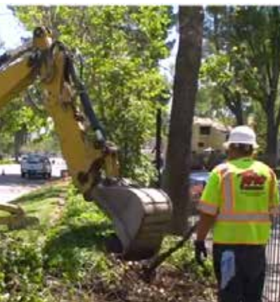
Construction of sidewalks
