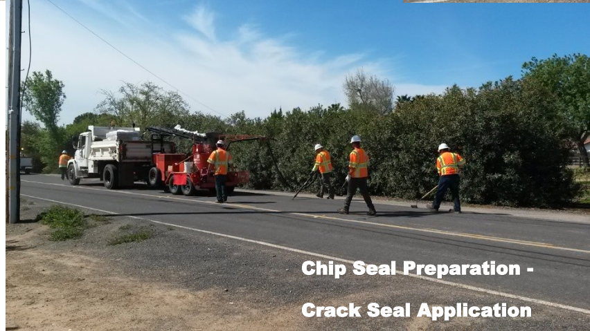
Chip Seal Preparation - Crack Seal Application
