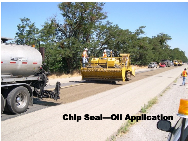
Chip Seal—Application of Chip Seal Rock on top of Oil
