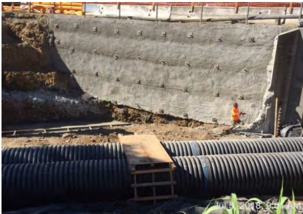
Stage 2 – Temporary Soil Nail Shoring
