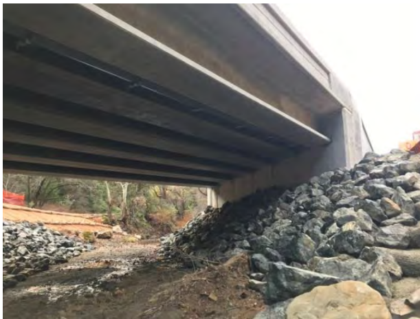
New Rock Slope Protection in Marsh Creek
