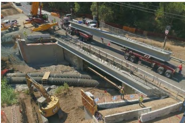
Stage 2 – Girder #2 Placement
