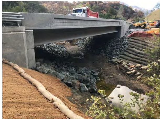
New Marsh Creek Concrete Girder Bridge
