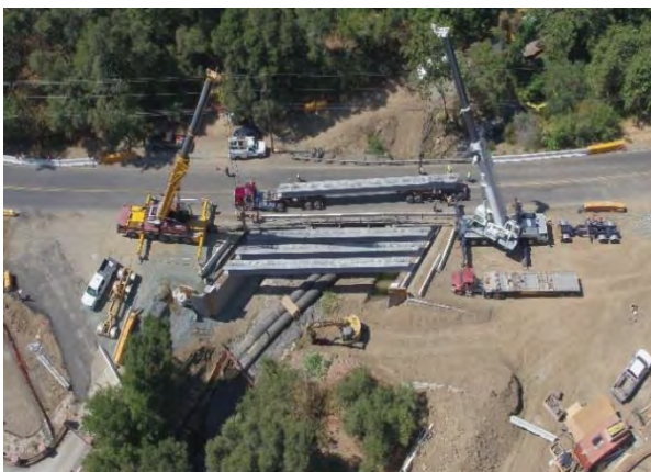
Stage 2 - Girder #4 Placement
