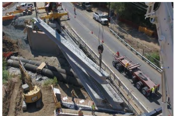
Stage 2 - Girder #3 Placement
