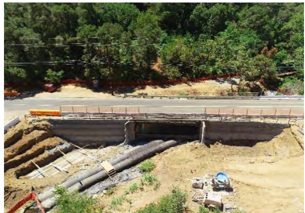
Stage 2 – Temp Soil Nail Shoring
