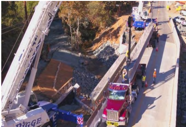
Stage 4 – Girder #6 Placement
