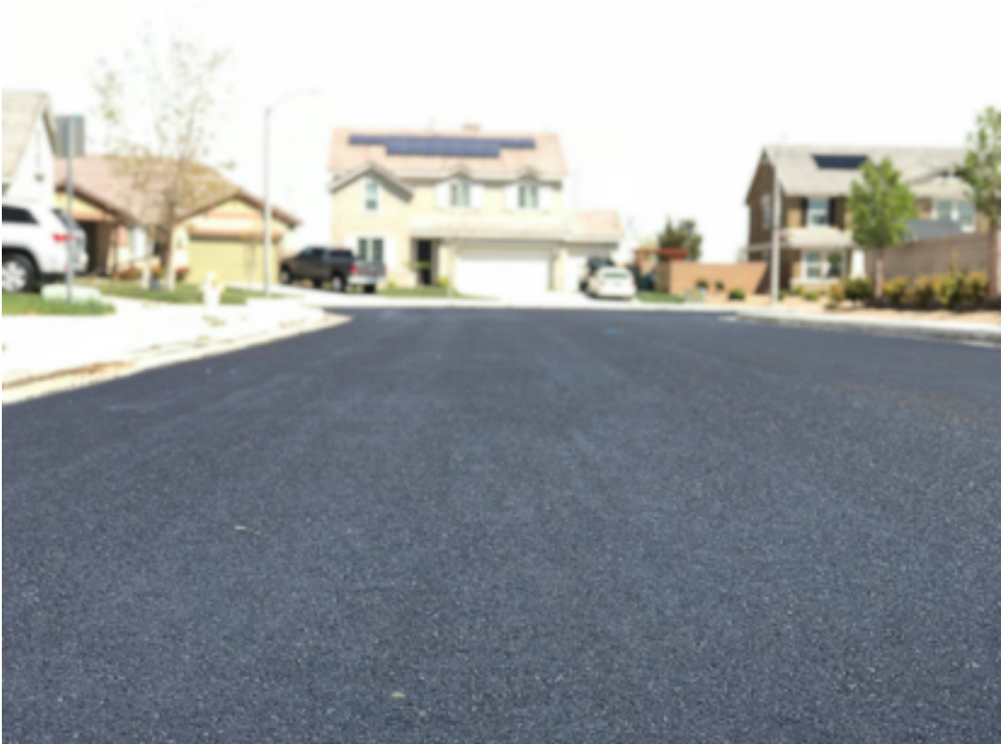
Neighborhood Fog Seal Project
