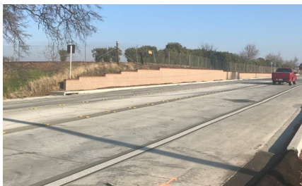
Atkinson Street after
