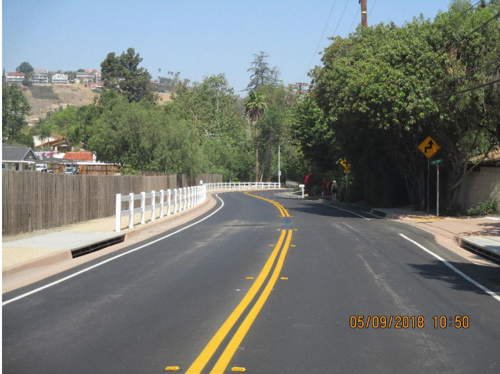
Project Completion – Roadway, Walking Path, Fencing, Storm Drain
