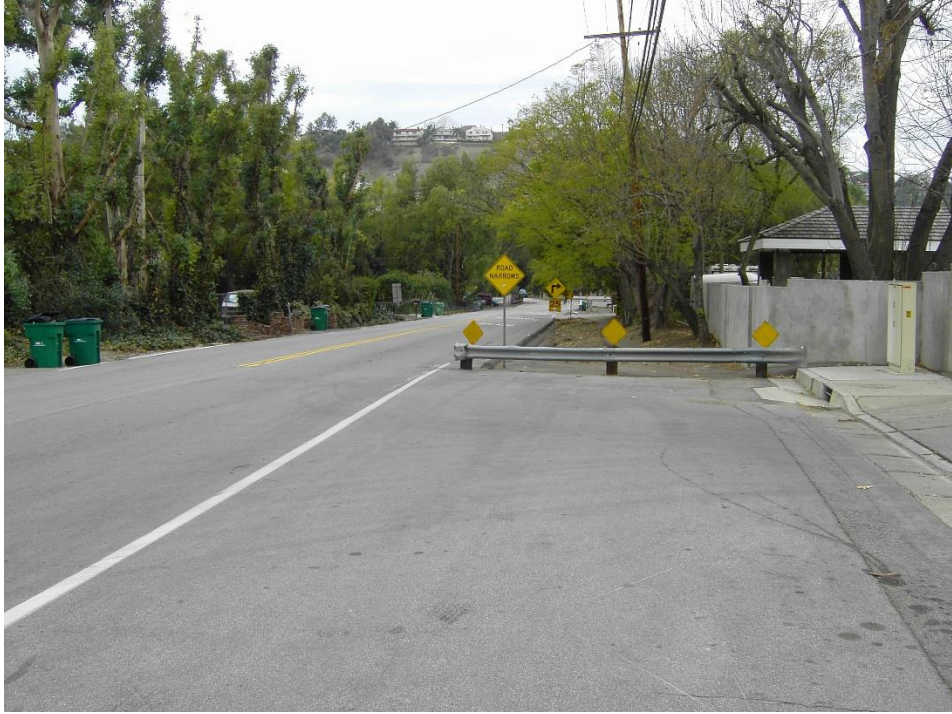
Pre-project condition with no safe route to school
