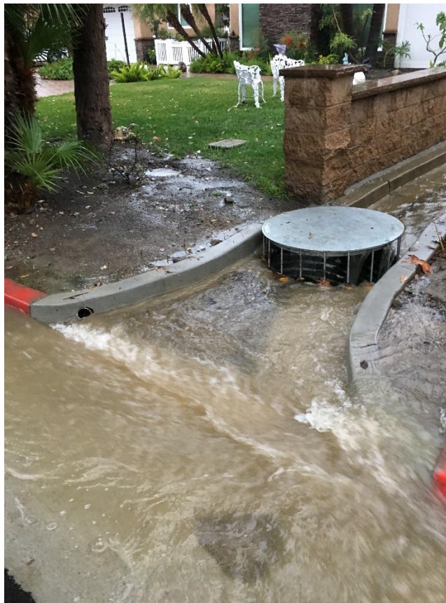
Project Completion – Newly Functioning Custom Catch Basin during storm event
