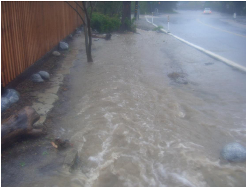
Pre-project flooding events
