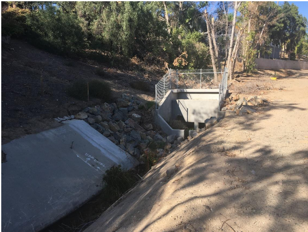
Project Completion – Weir Outlet structure
