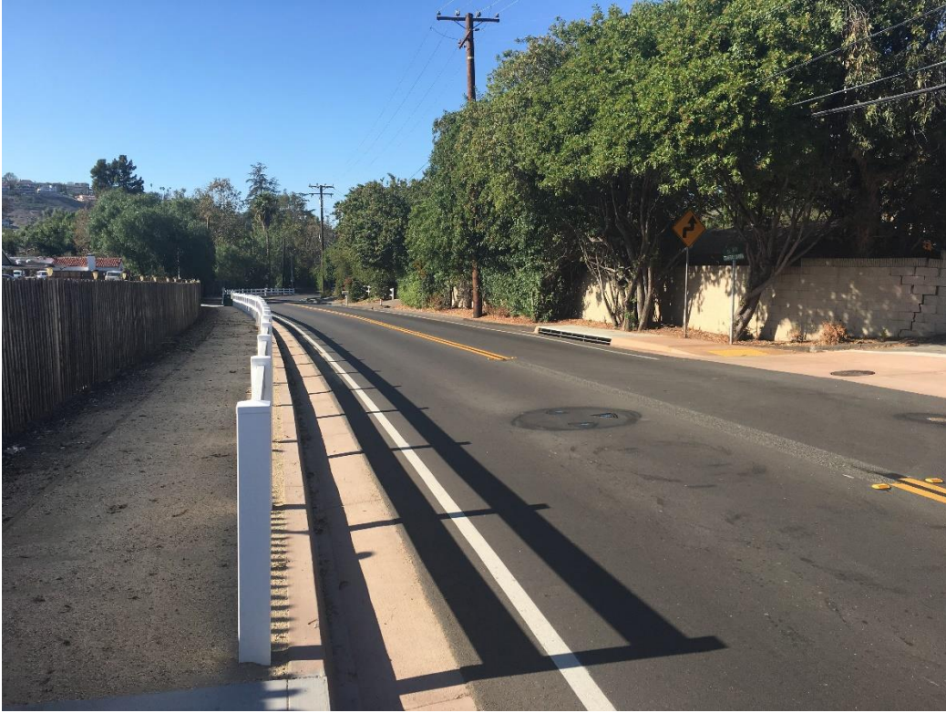
Project Completion – Roadway, Walking Path, Fencing
