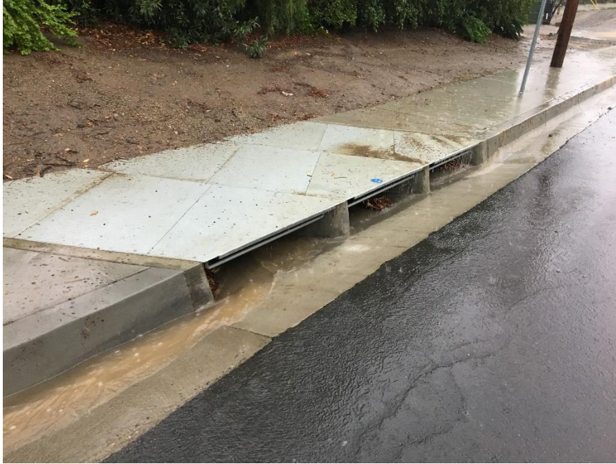
Project Completion – Newly Functioning Custom Catch Basin during storm event
