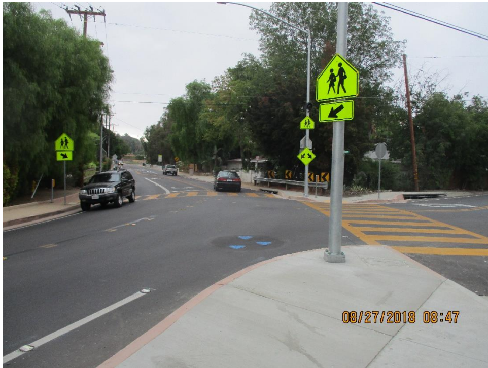
Project Completion - Barrett Lane/Crawford Canyon Intersection
