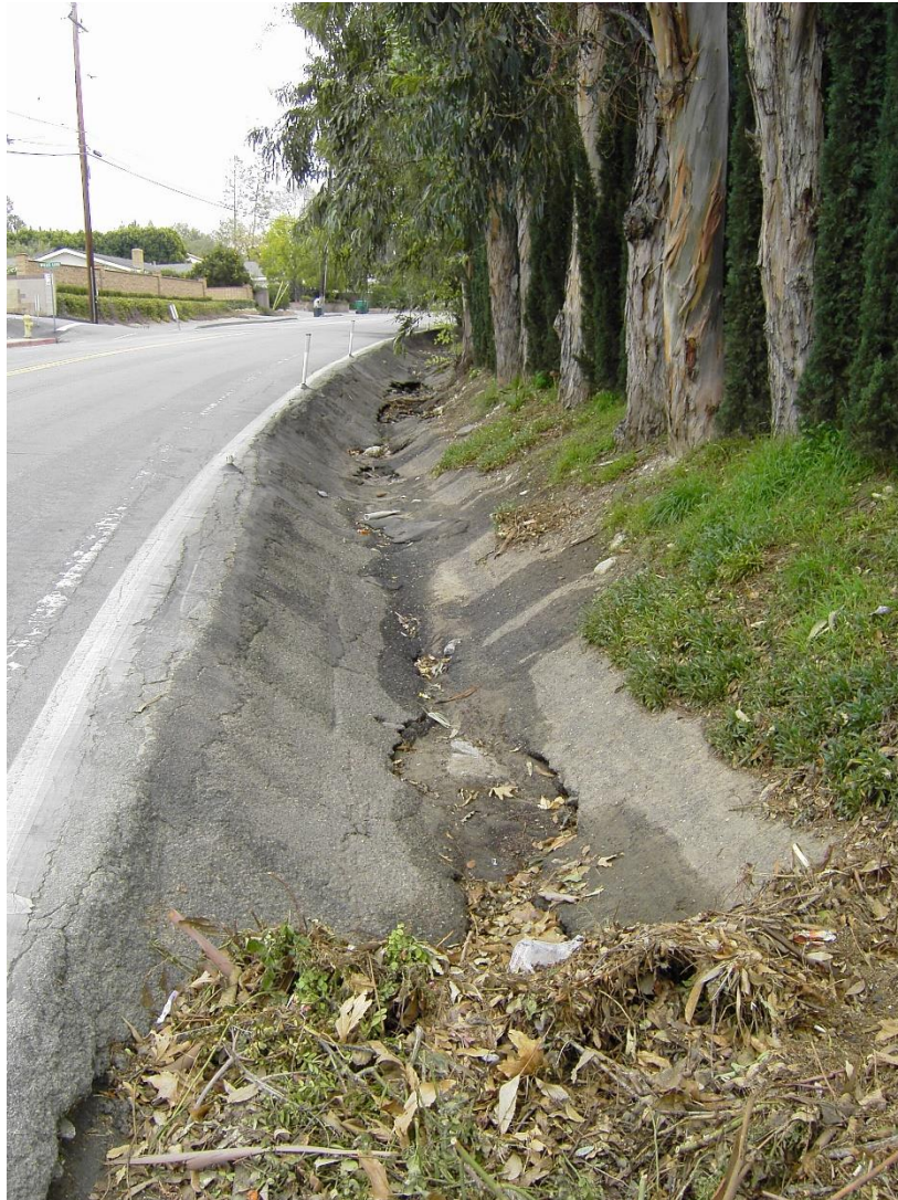
Pre-project condition with V-ditch
