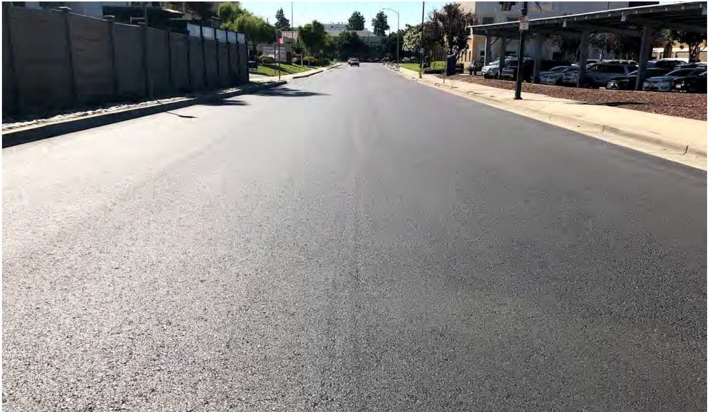
LUDLOW WAY (AFTER)
