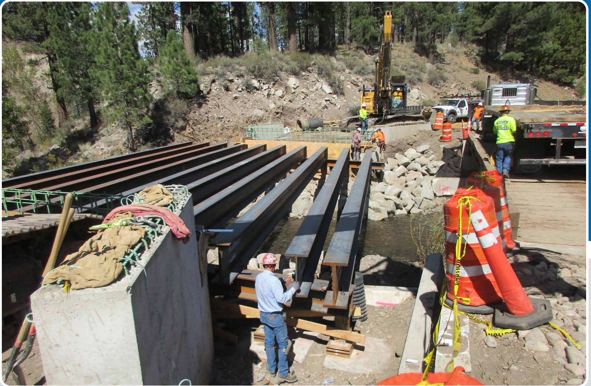
Single-Span Falsework DIXON MINE ROAD BRIDGE OVER WOLF CREEK, ALPINE COUNTY, CA
