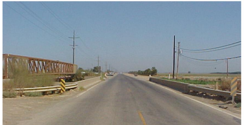
Before: Russell Avenue bridge in a 2006 photo.
