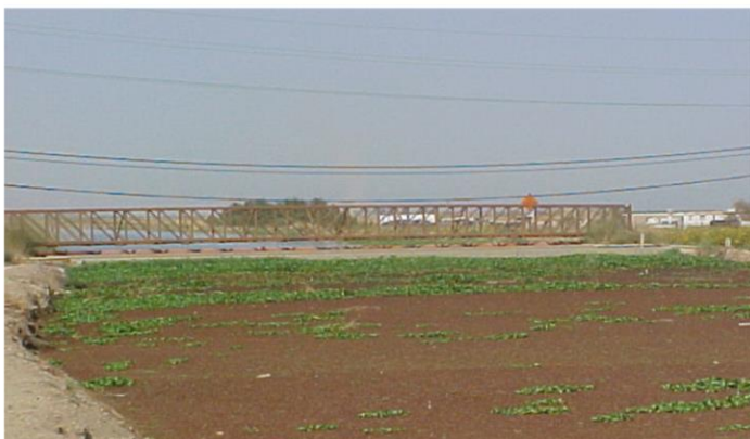
Before: Outside Canal looking west at the east side of the Russell Avenue bridge.
