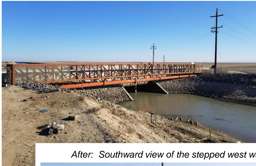
After: West side view of the new double box culvert at low water levels.
