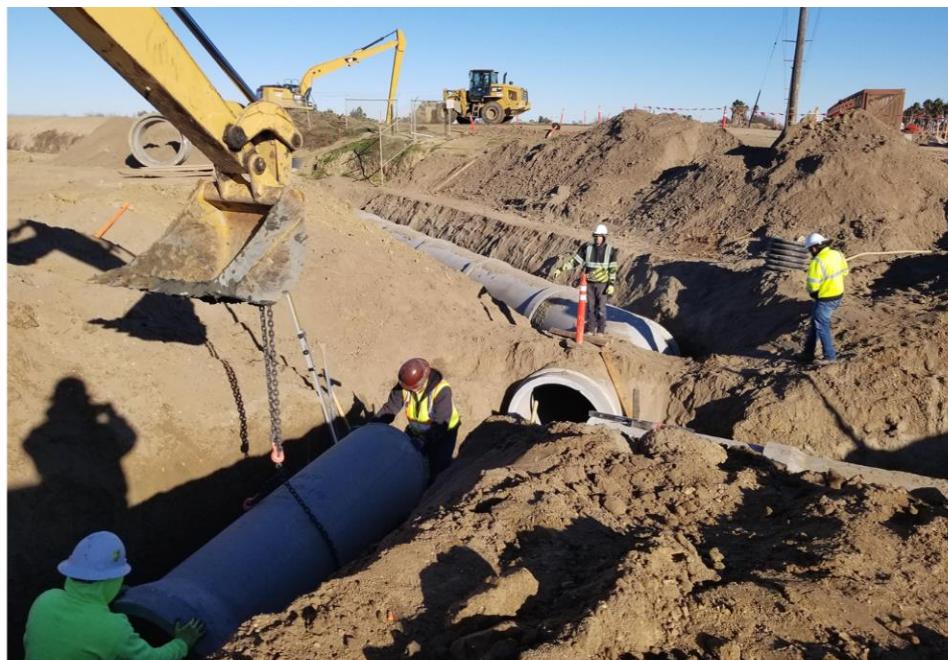
Reinforced concrete pipe installation in February of 2020.
