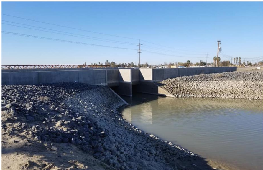
After: East side view of the new double box culvert at low water levels.
