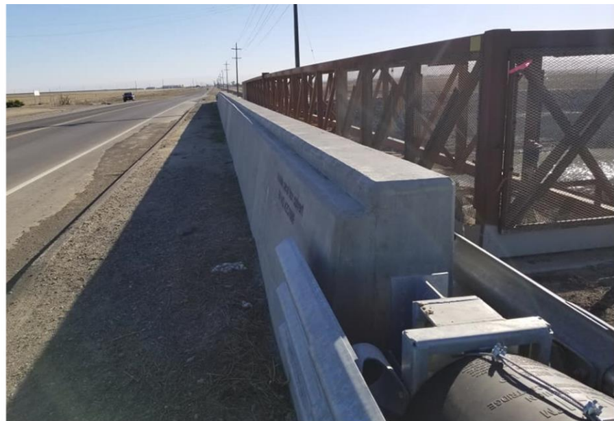
After: Southward view of the stepped west wall.
