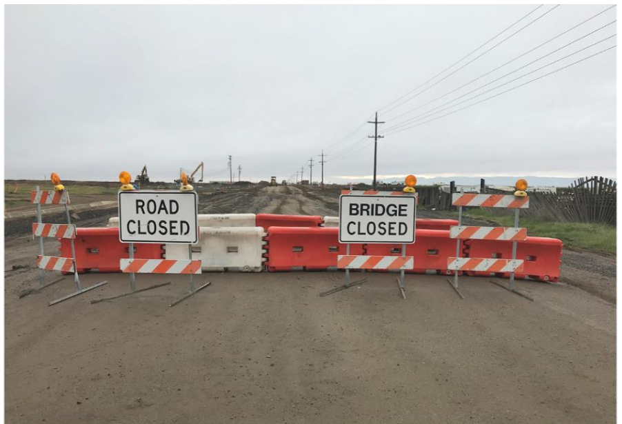
Road closure signs seen in place throughout the project.
