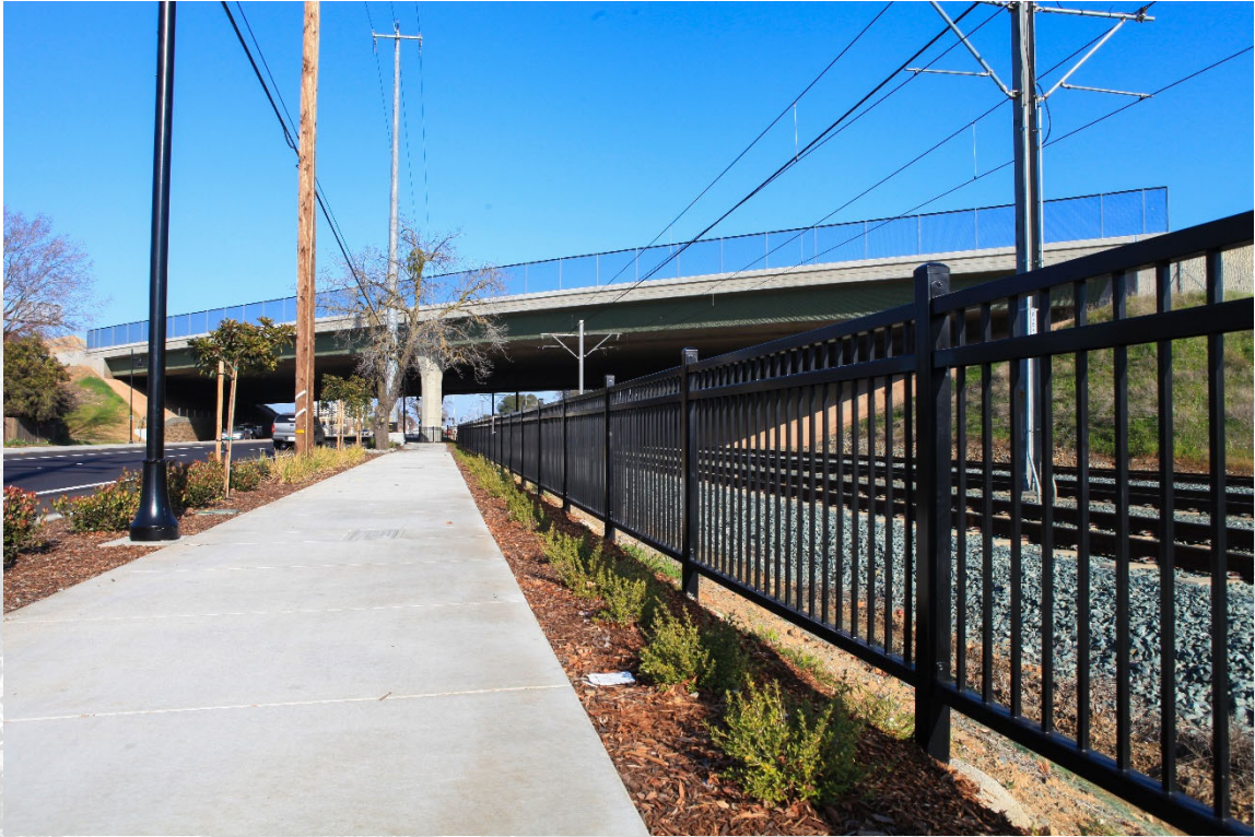
Sidewalk and Decorative Fence Approach US-50 Undercrossing
