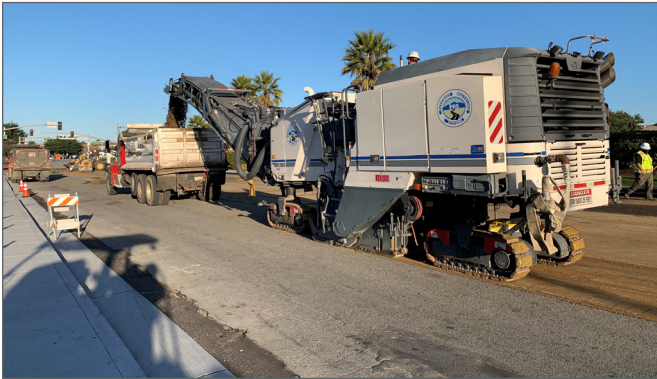
Westbound - Asphalt being milled for reclamation
