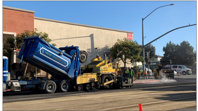
Eastbound - Reclaimed asphalt being mixed, poured, and compacted
