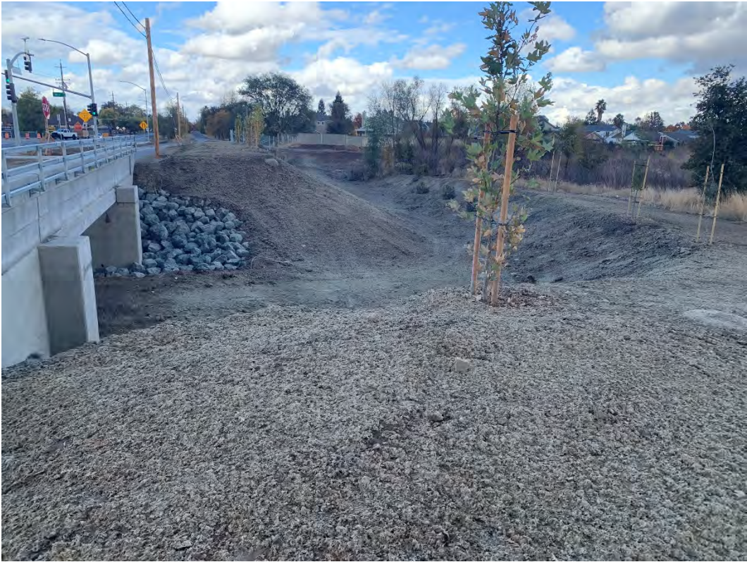
Completed Magpie Creek and rock slope protection
