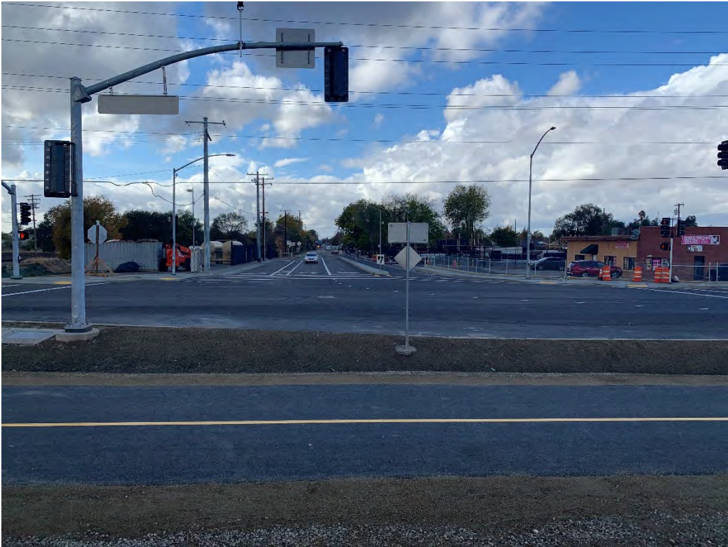
Completed Rio Linda Boulevard and Main Avenue Intersection facing west
