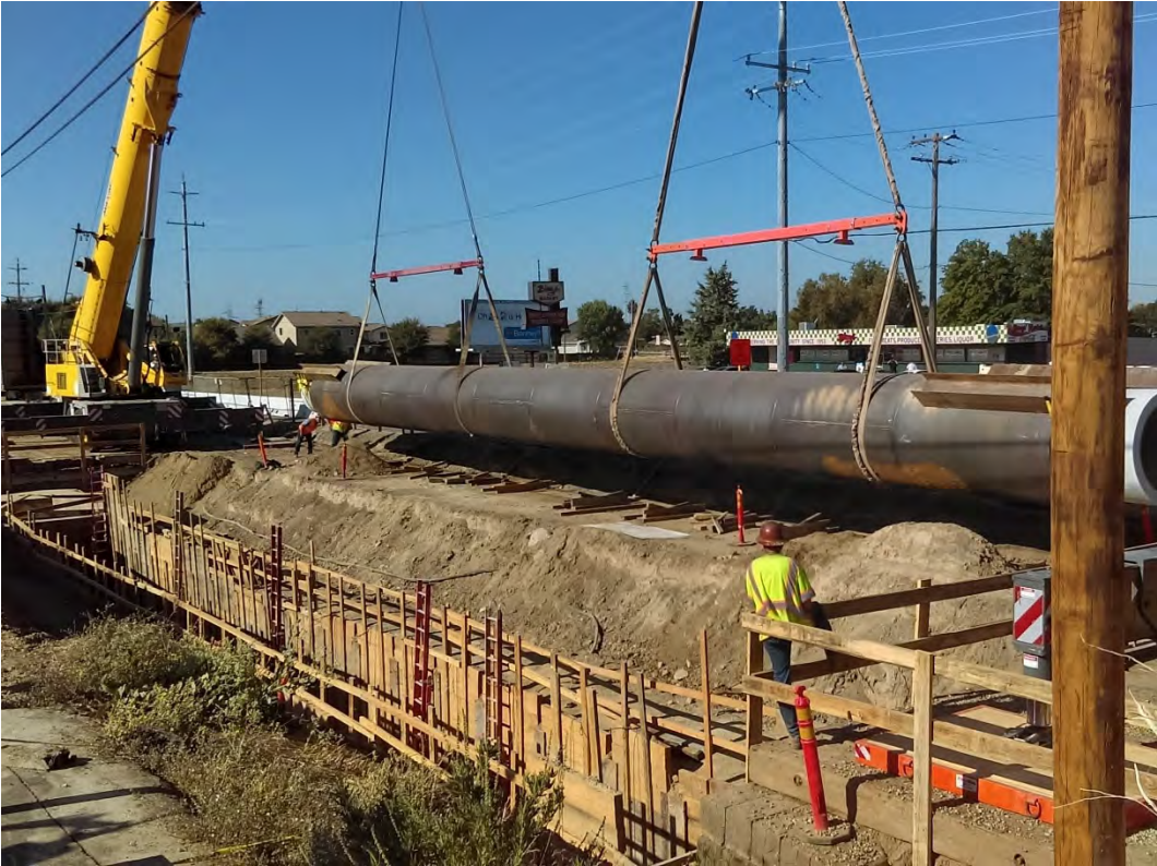
Installation of sewer casing and pipeline
