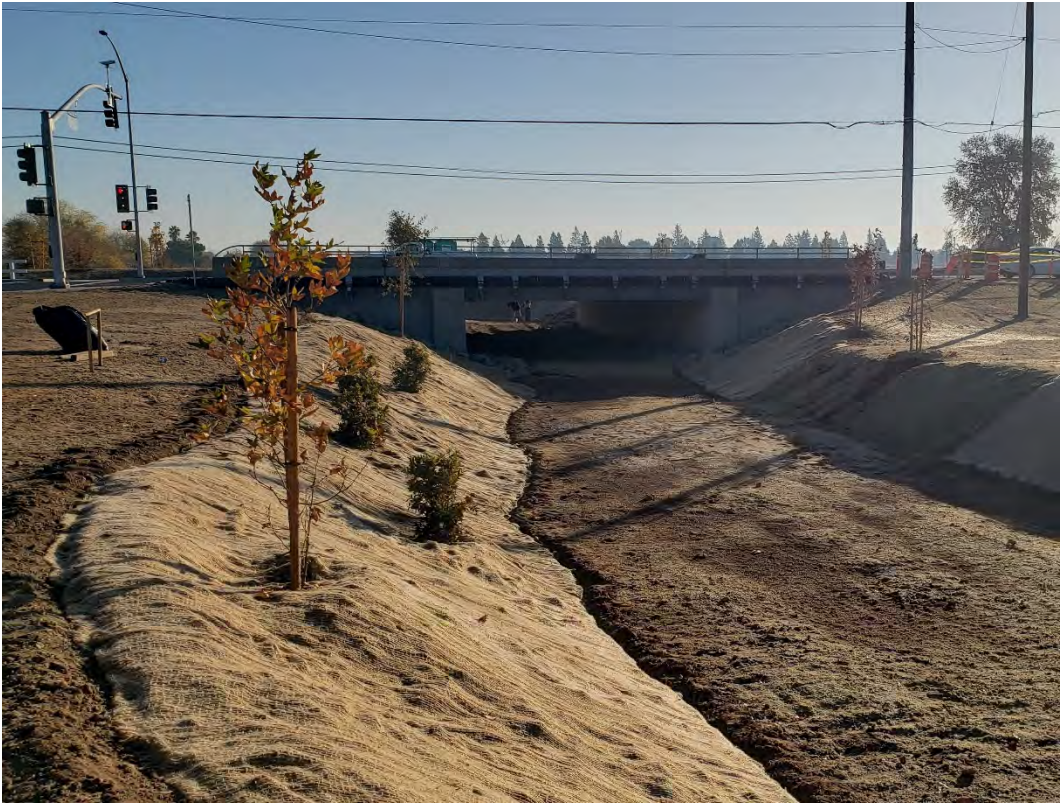
Complete bridge replacement and Magpie Creek enhancements
