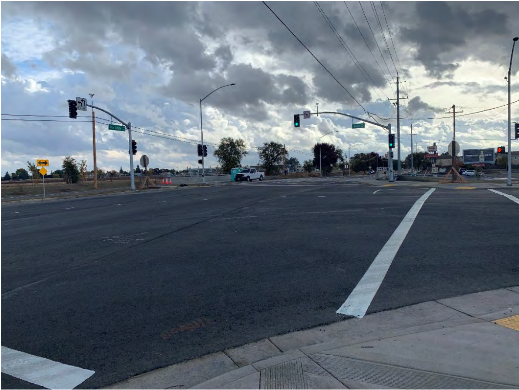
Completed intersection improvements facing south on Rio Linda Boulevard
