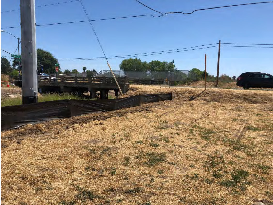
Beginning of construction and existing Rio Linda Boulevard Bridge
