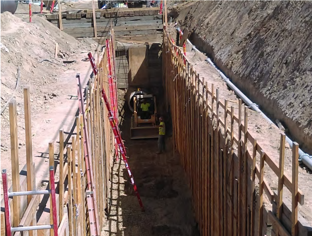
Initial grading of utility trench
