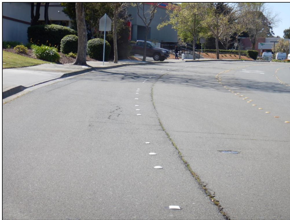
Figure 2.7 Example of Local Street with PCI of 66
