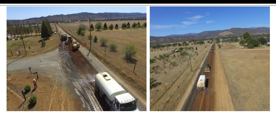
The roadway pavement section was reconstructed the using Full-Depth Reclamation (FDR) with an asphalt overlay, corrections to roadway cross-slopes, and shoulder drainage improvements. FDR saved the County 19% in construction cost when compared to other potential solutions.
