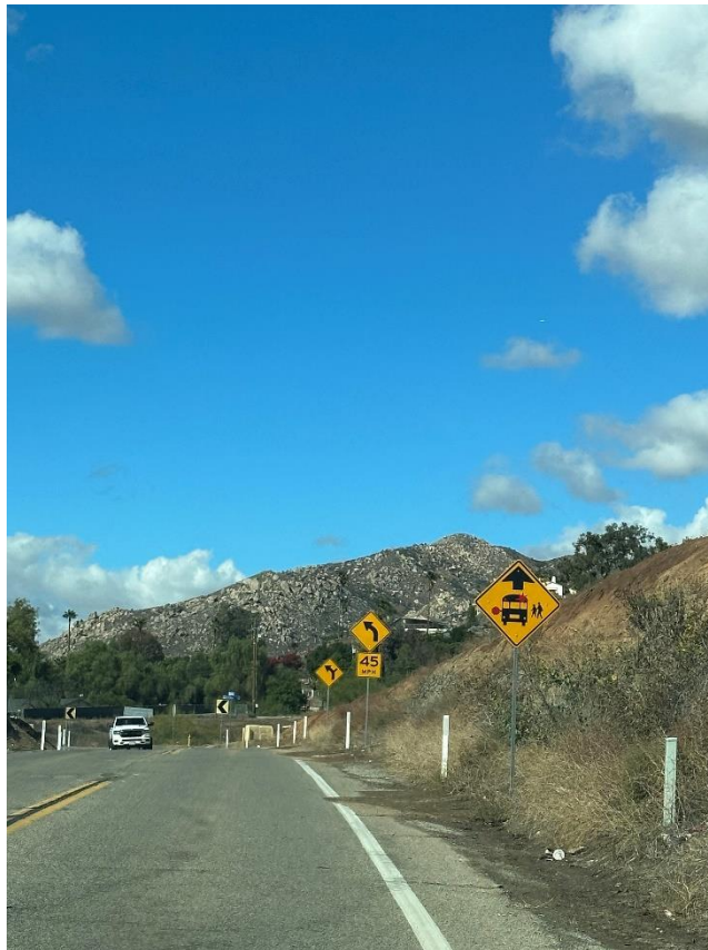
Figures 5, 6 and 7. Shows post construction signs installed as well as new striping.
