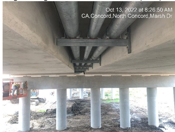
PG&E hanger and brackets installed under the 3' closure pour section
