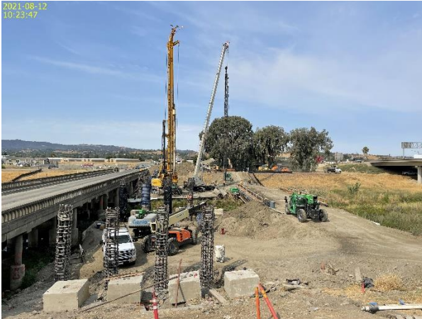
Stage 1 bridge foundation construction (CIDH) (8.12.21)
