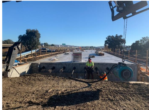
Stage 1 bridge deck post – tensioning (10.28.21)
