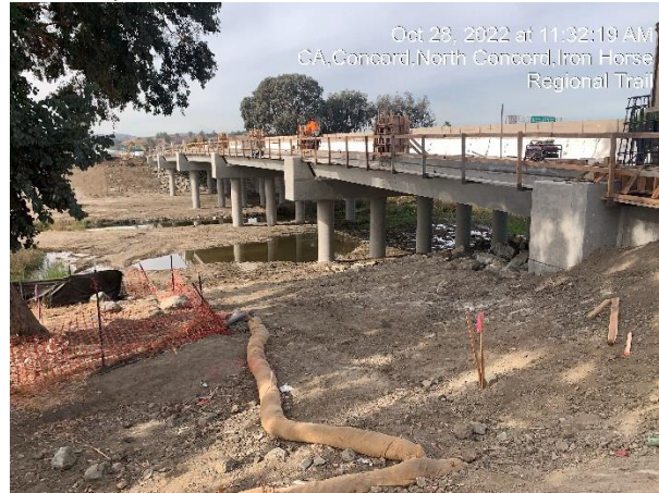
South side view of the new bridge face West (10.28.22)
