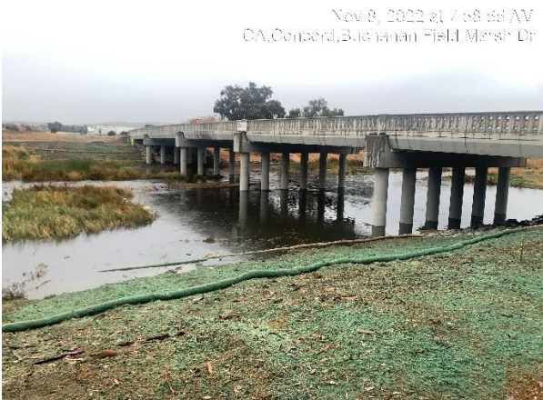
North side view of the new bridge face East (11.8.22)
