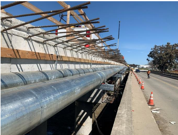
Stage 1 PG&E hanger and brackets installation (3.18.21)
