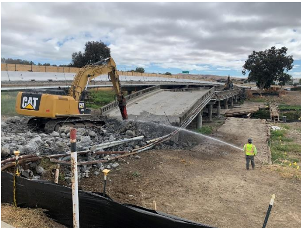
Stage 2 old bridge demo (7.5.22)
