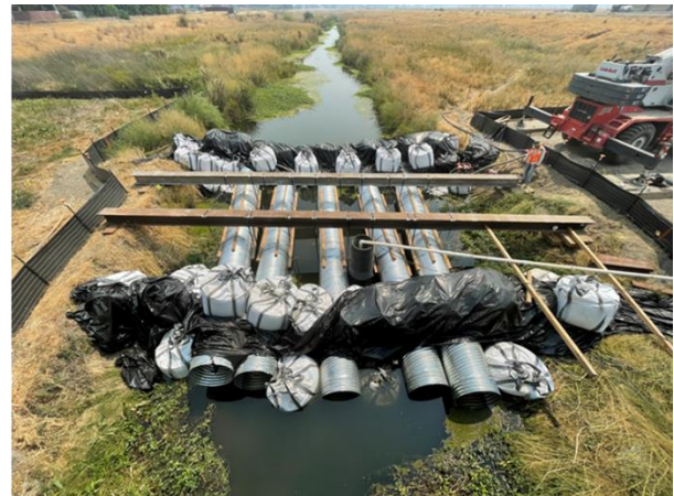
Stage 1 creek diversion system installation (8.31.22)
