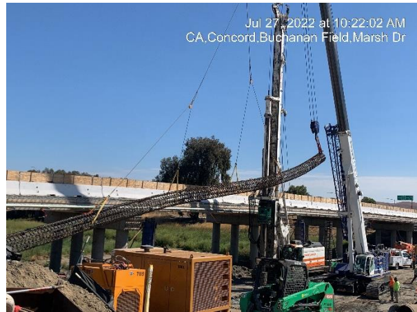
Stage 2 bridge foundation construction (CIDH)
