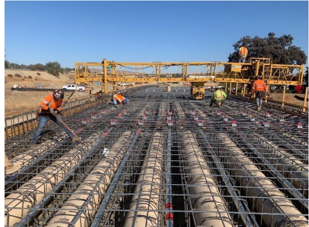
Stage 1 deck falsework and Sono-voids placement (9.15.21)
