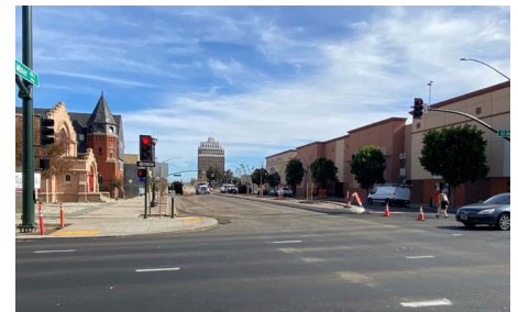
2021 during construction phase.
