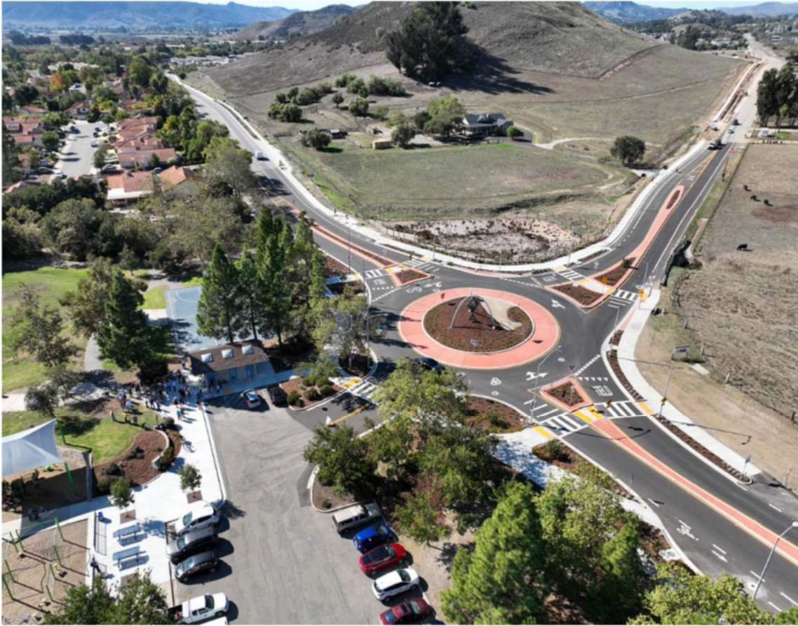
Aerial view of the completed roundabout
