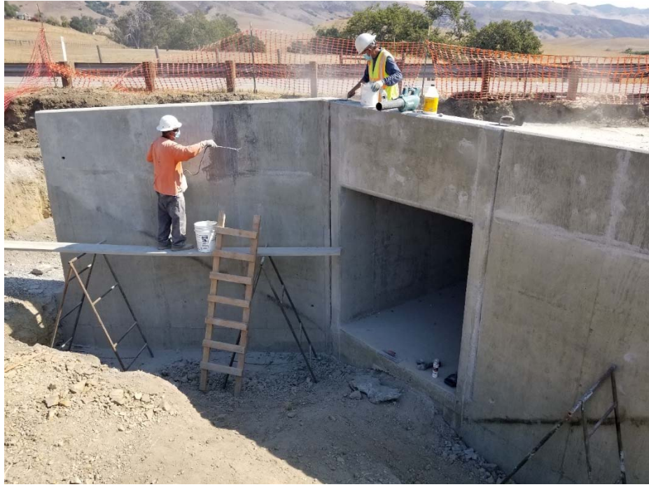
Construction of culvert crossing Orcutt Road
