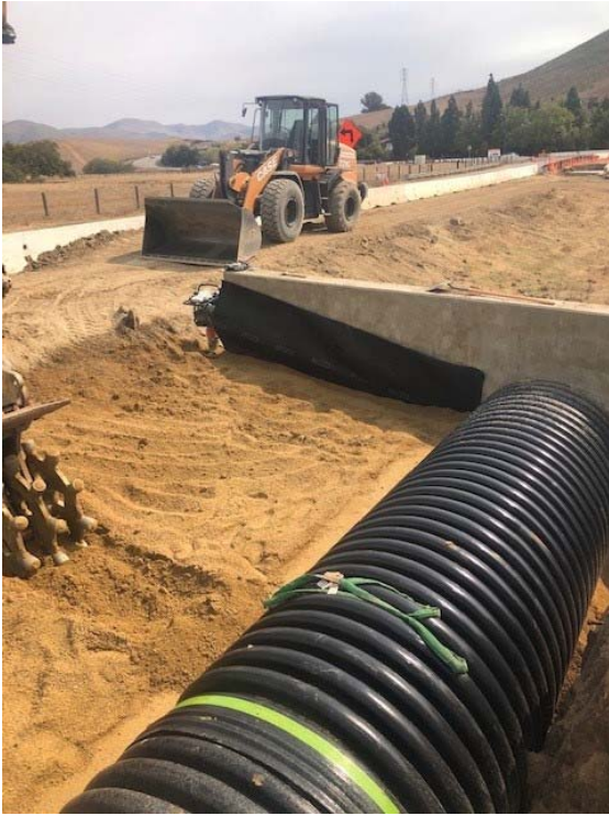
Construction of private driveway culvert
