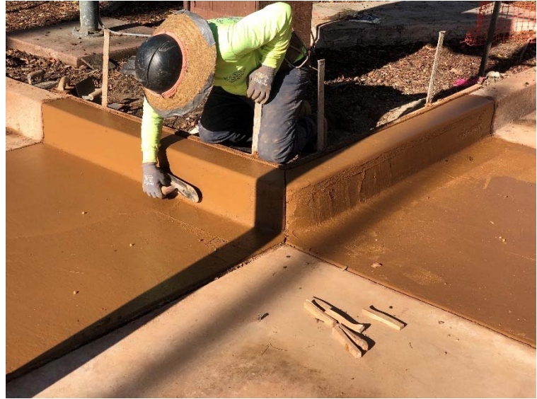
Construction of new sidewalk panels
