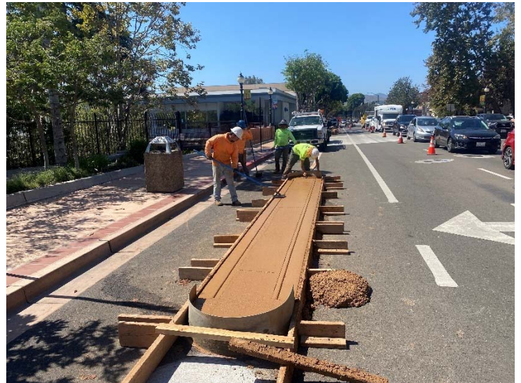
Construction of concrete bike lane median
