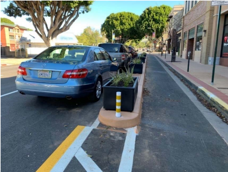
Completed parking protected separated bike lane on Marsh Street with planter boxes
