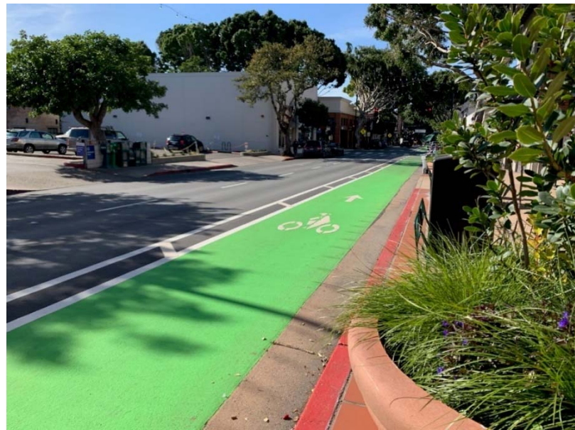
Completed green buffered bike lane on Higuera Street
