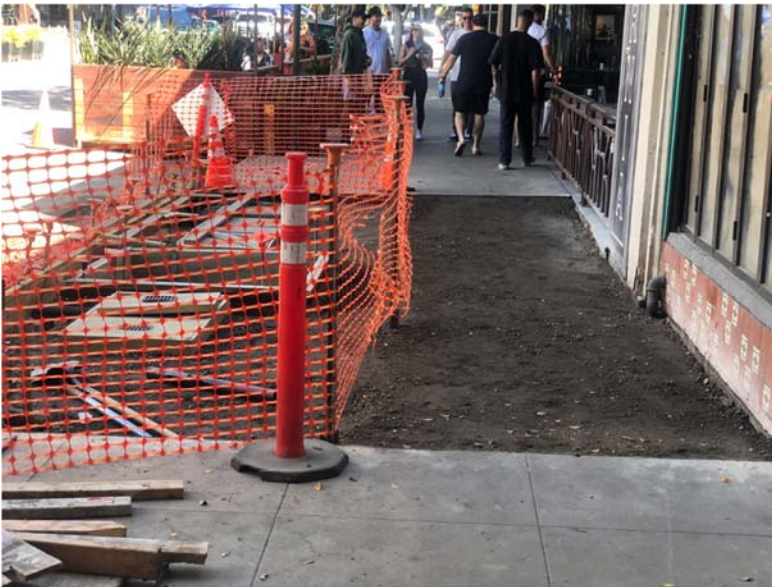
Temporary accessible path during construction
