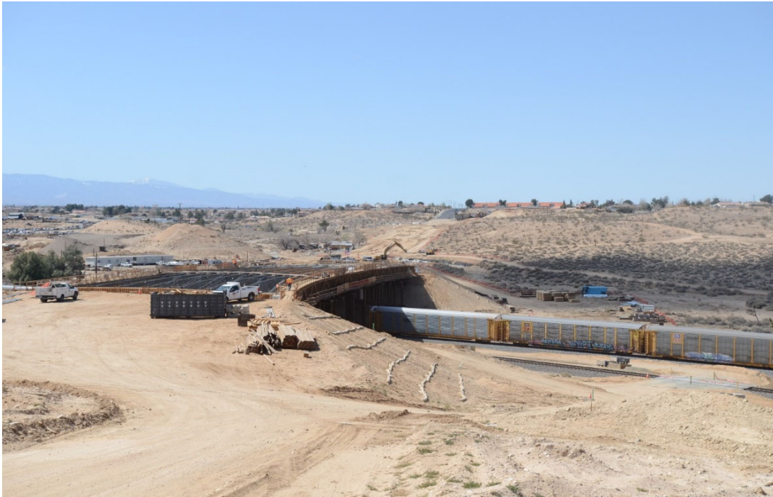
False work and reinforcing bars in place.
