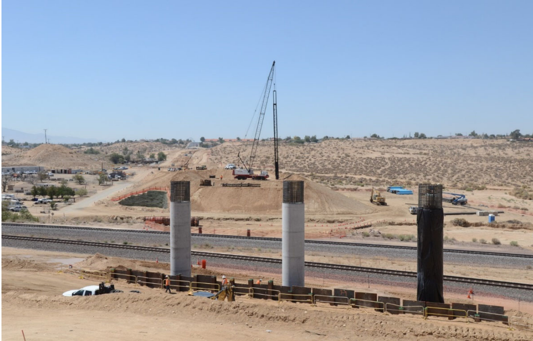
One set of columns poured and working on the second set.
