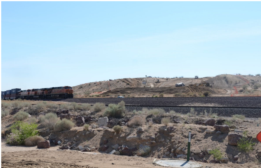
Slowly removing soil from hill of future alignment.
