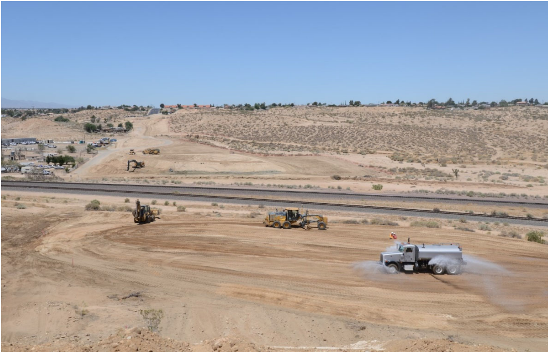
Start of the earth work operation for the bridge.
