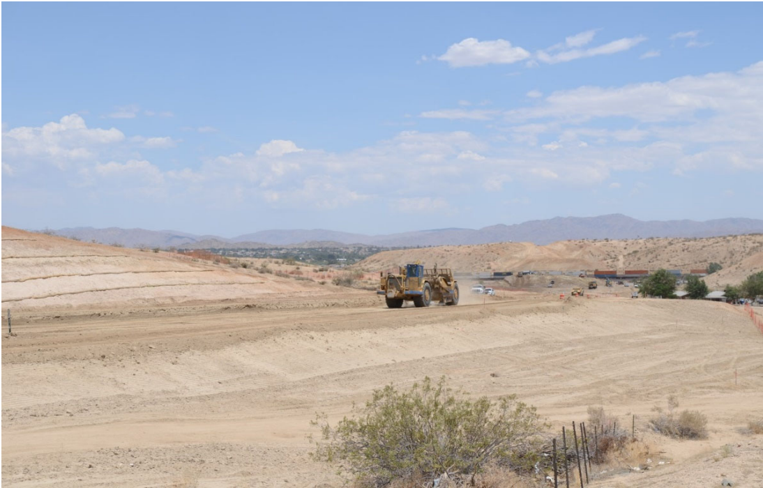
Filling on the future roadway
