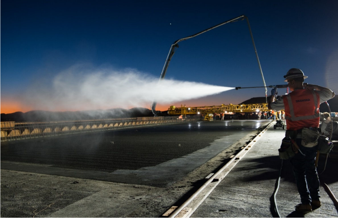
Spraying curing compound on the surface of bridge
