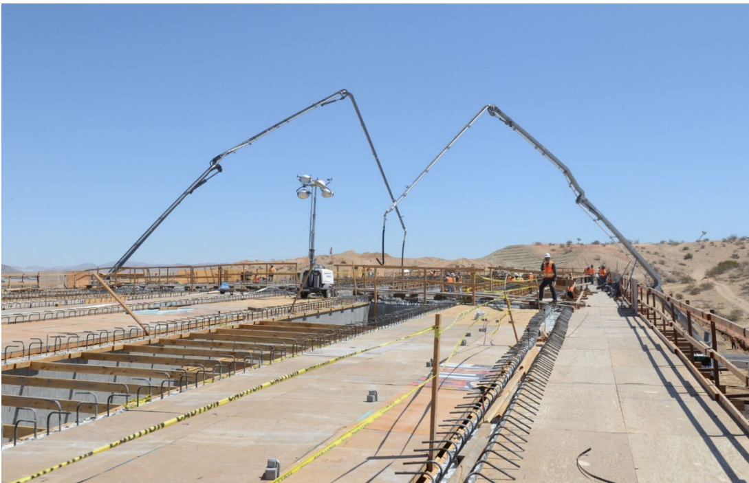
Placing concrete for the bridge deck
