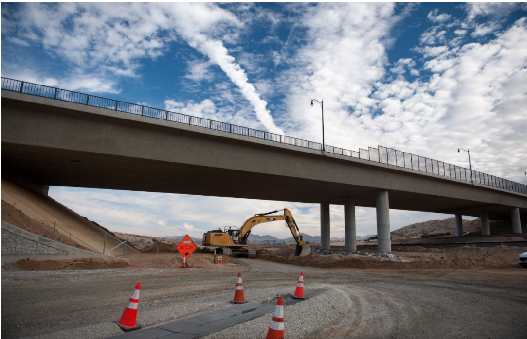
Restoration of the wash under the bridge
