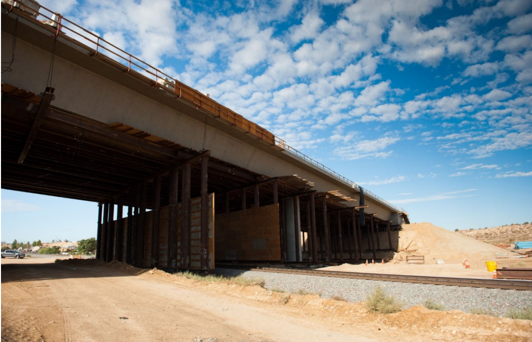
Removal of the false work after concrete has been stressed
