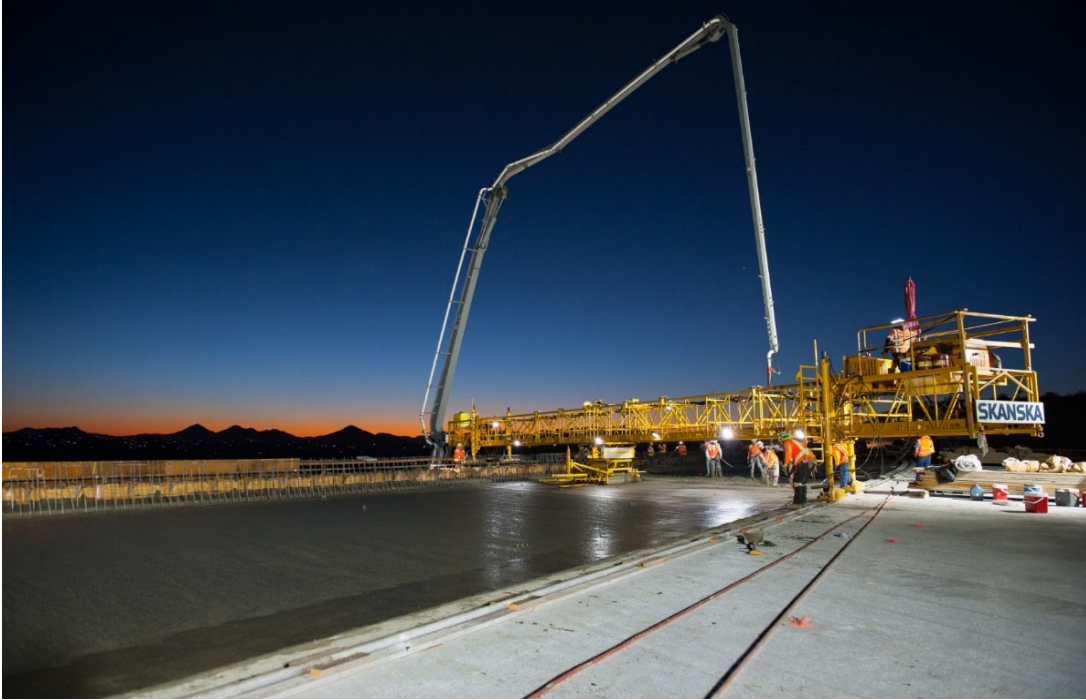
Screeding the concrete deck of the bridge
