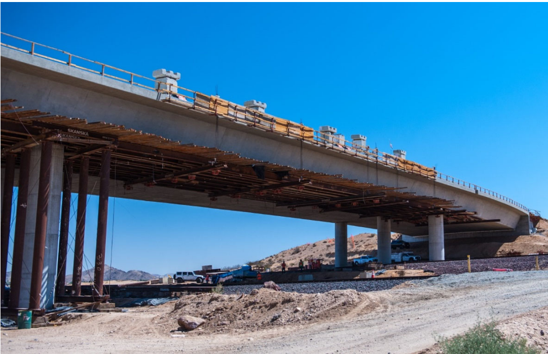
Removing the falsework over the rail road with a track closure.
