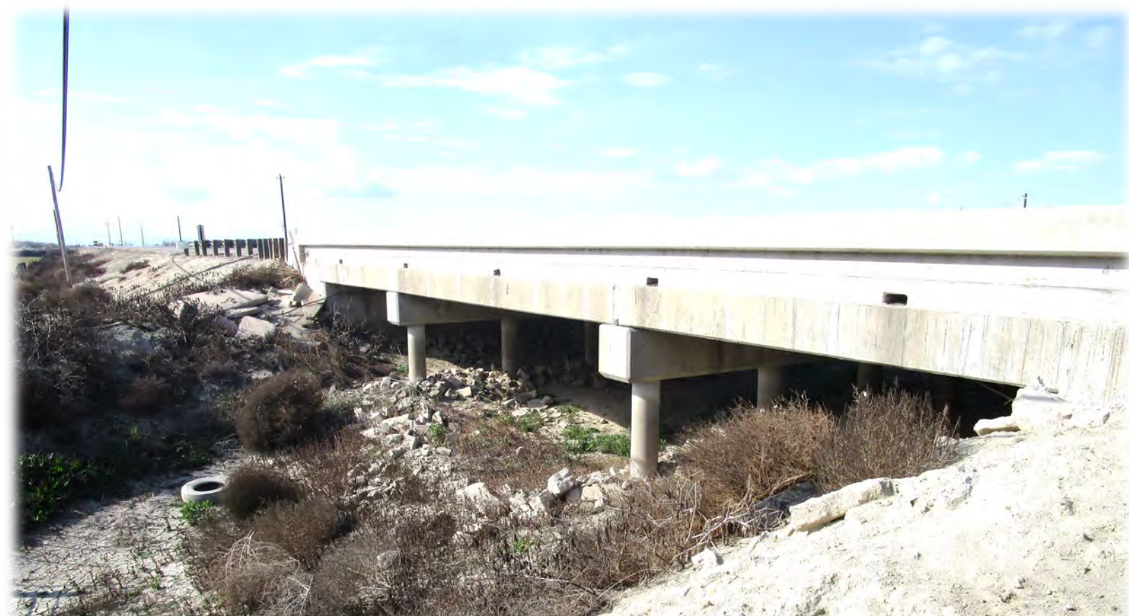
The old eastern bridge on Manning Ave over James Bypass.
