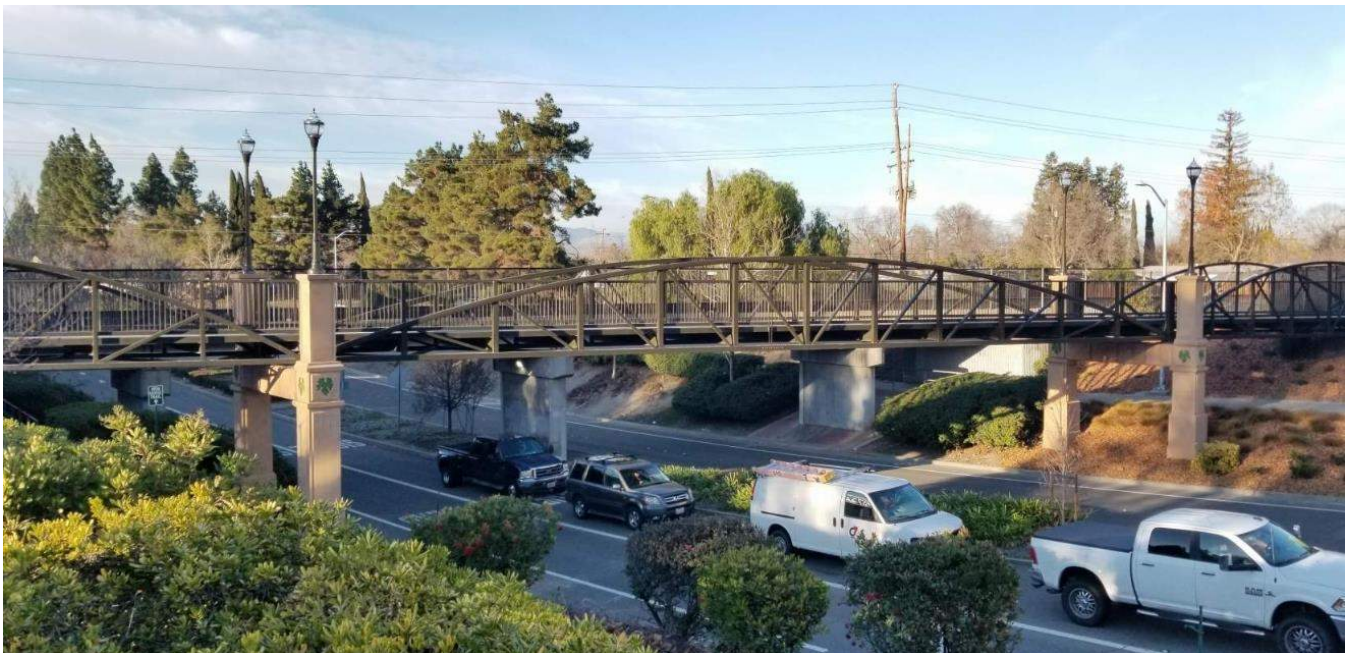
Iron Horse Trail - Murrieta Blvd Trail Bridge Crossing
