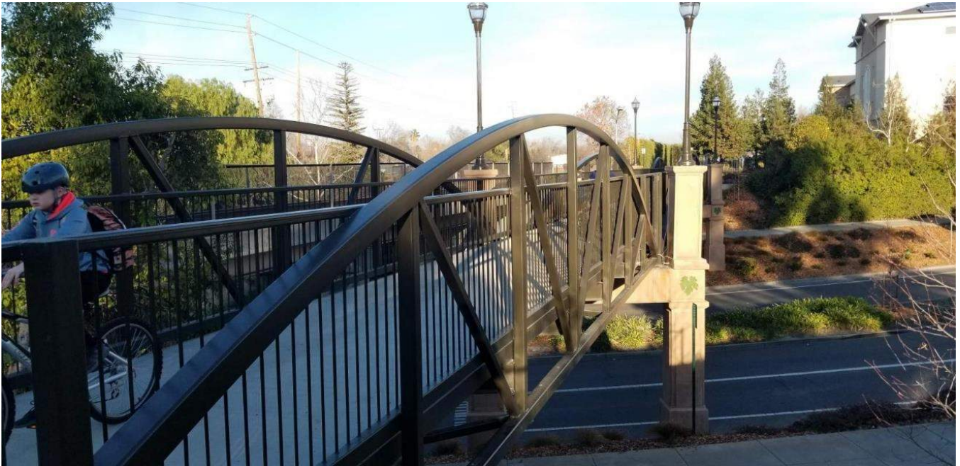
Iron Horse Trail - Murrieta Blvd Trail Bridge Crossing
