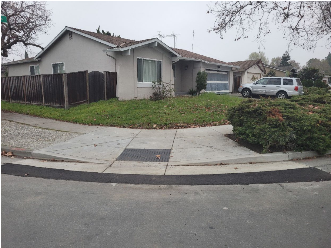
Finished curb ramp that meets current ADA standards.
