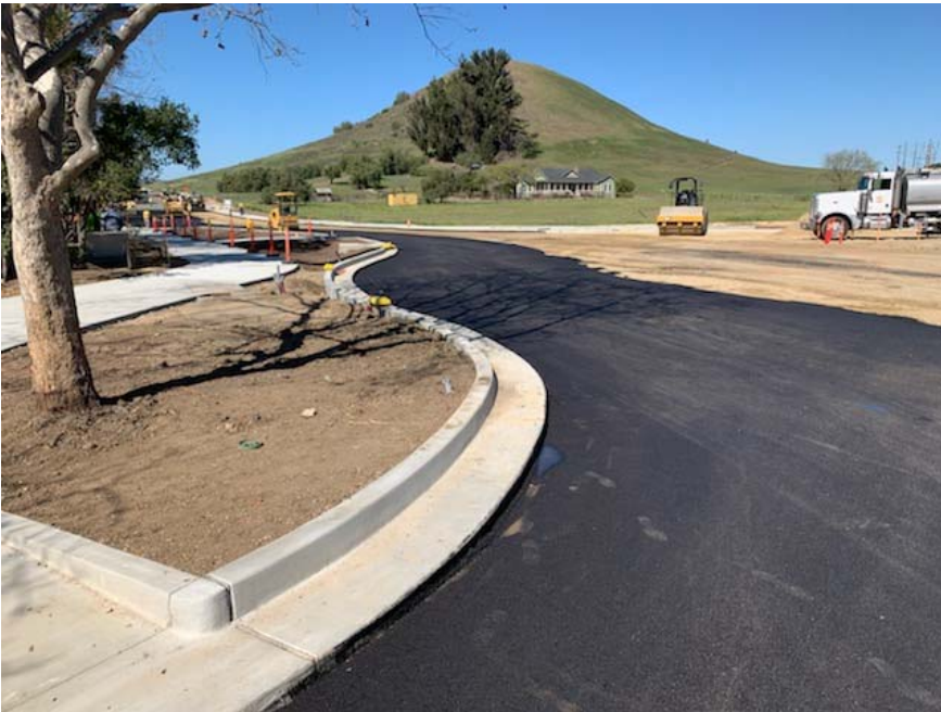
Roadway construction of roundabout
