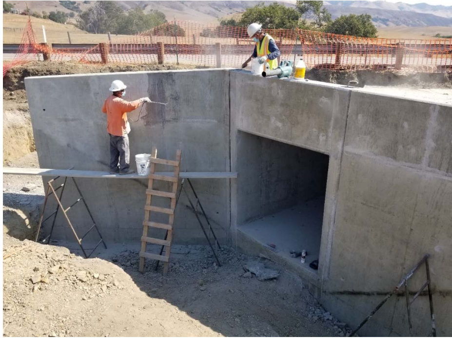
Construction of culvert crossing Orcutt Road
