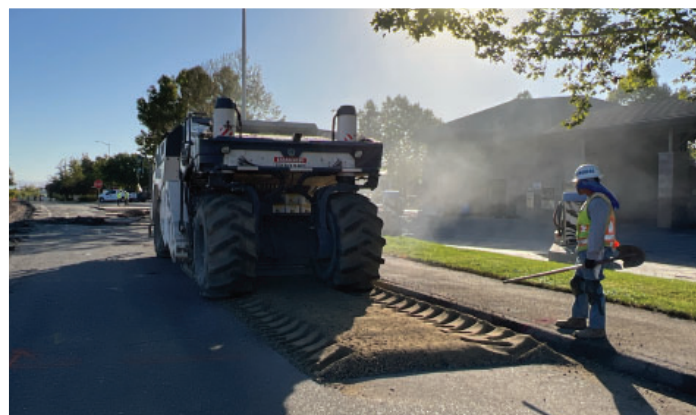
Full Depth Reclamation
