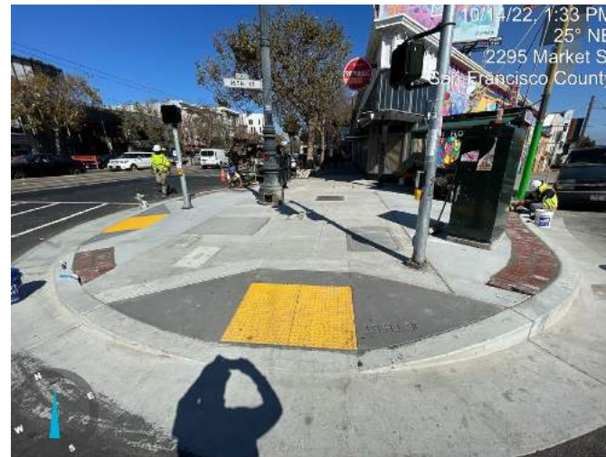
Pedestrian bulb-out with 'Path of Gold' light fixture upgrades and brick paver border
