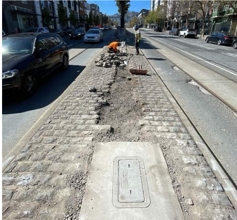
Cobblestone median installation
