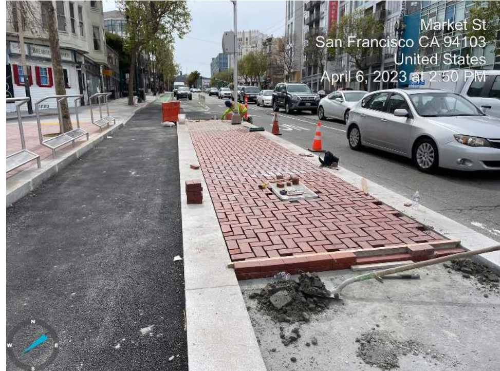
Paver median installation with granite curbs
