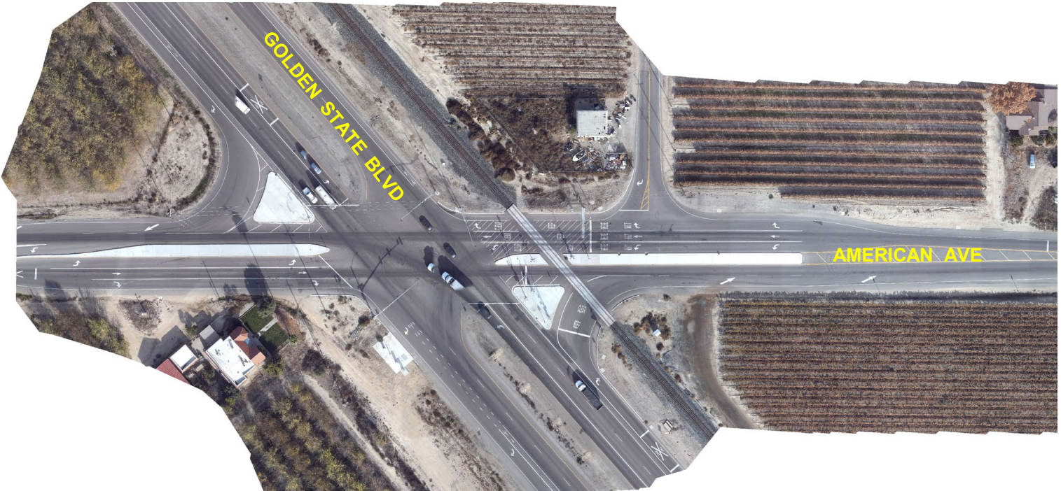
Aerial survey of the finished intersection
